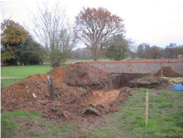
DP 1. Area of proposed swimming pool. Looking east-south-east.
