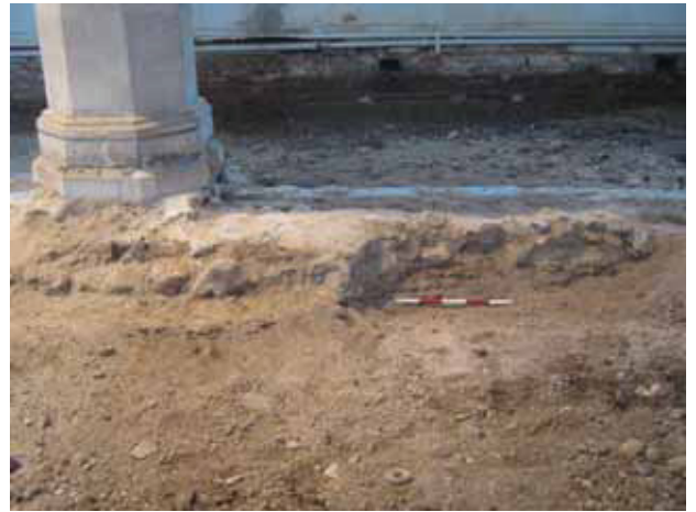
14 Wall Foundation M2027. Looking N
