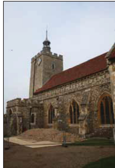
2 Felsted church. Looking North-West
