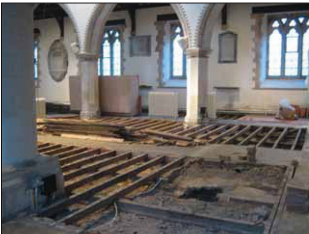
3 Existing modern floor within the nave. Looking North-West
