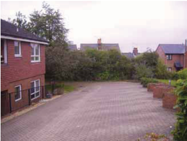
DP 7 Extensive area of block paving located to the south of St Andrew's Place and within the site's northern section, formerly used for resident's/visitor car parking
