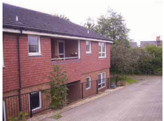
DP 8 Northern frontage of St Andrew's House comprising a two storey, red brick built building partially cut into the natural ground level, view west-north-west
