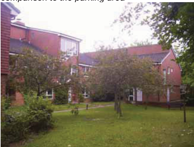
DP 11 Western frontage of St Andrew's House comprising a red brick built building ranging over three storeys, view south-east
