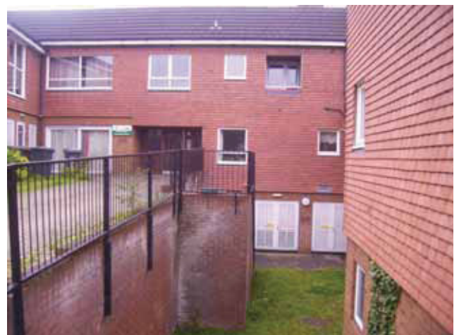
DP 6 Area of extensive groundworks and high brick retaining wall in the centre of the site depicting the lower level of St Andrew's House
