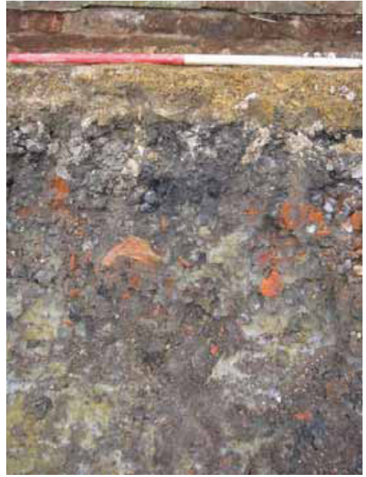
2 Sample Section. Northwest end, looking northwest.
