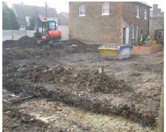
6 General site photograph. Looking south.
