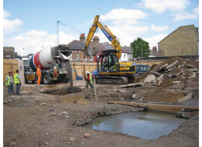
DP 8. Groundworks in progress. View NE.
