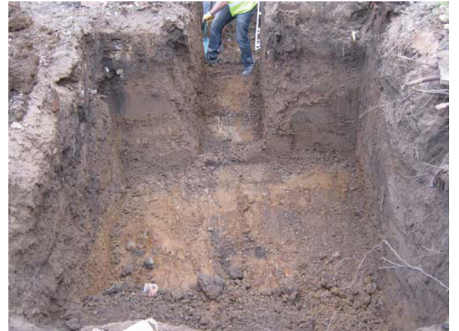
DP 4. W foundation trench. View N.
