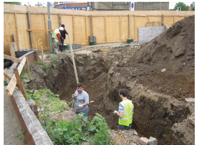
DP 6. NW foundation trench. View NNE.
