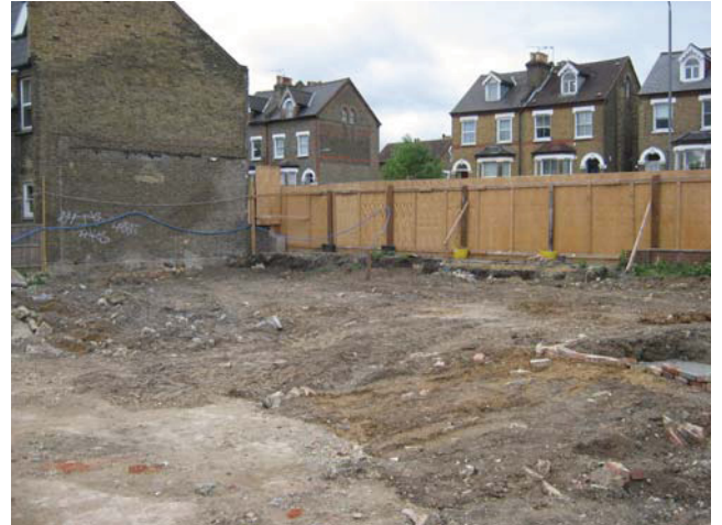
DP 2. W part of the site. View SW.
