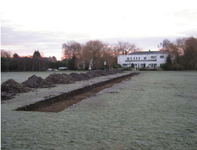
DP 1. The site. Looking south-south-east.
