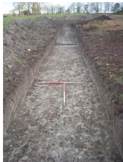
12 Trench 6. Looking South.
