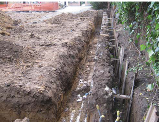
DP 5. S foundation trench. View ENE.
