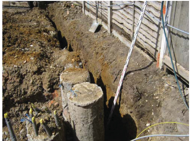
DP 2. N foundation trench. View NW.
