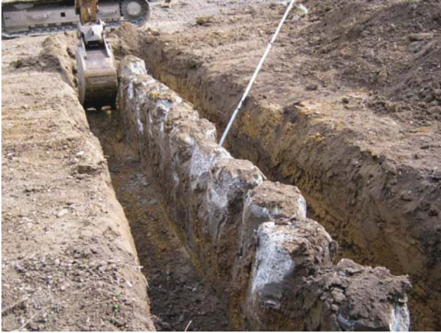
DP 7. W foundation trench. View NE.
