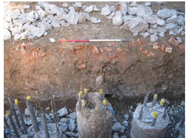
DP 4. E foundation trench. Sample section 1. View WNW.
