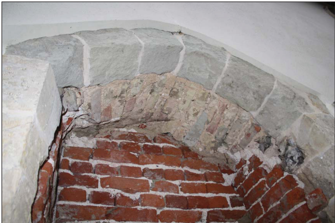
Plate 4 Arch soffit on the blocked doorway on the north side of the chancel, taken from north (DP 13)
