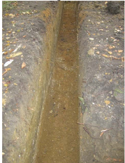
10 Fully excavated footing trench. Looking east.
