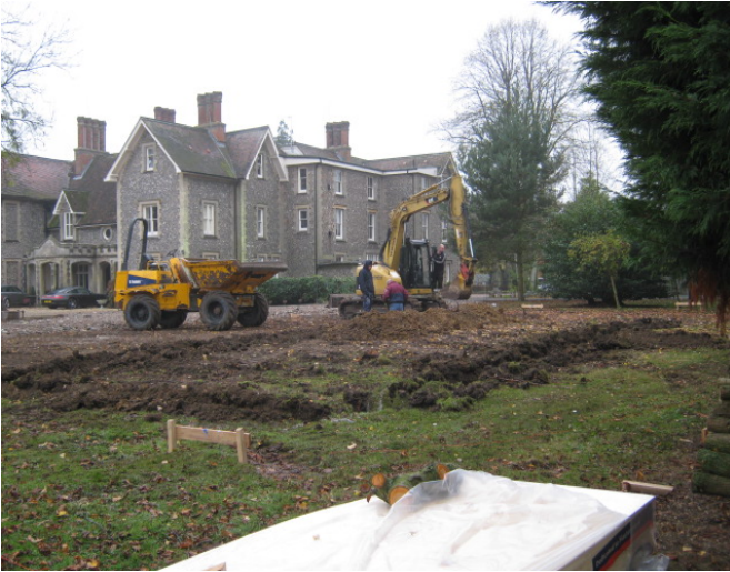
1 General view with Rowney Priory in background. Looking southwest.
