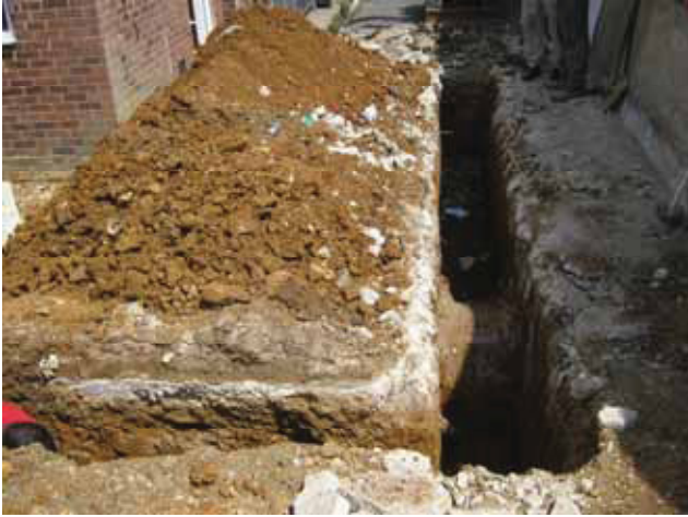
DP 7. S rear/side foundation trench. View E.
