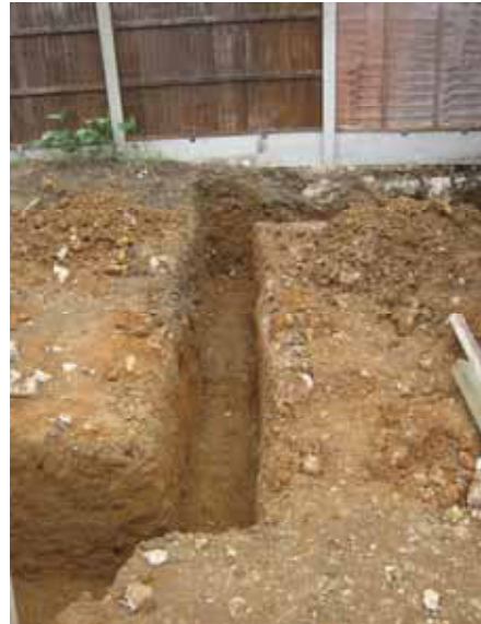
DP 4. W foundation trench, N part. View N.
