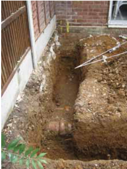
DP 3. N foundation trench. View E.
