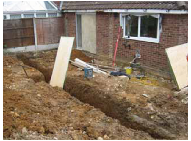
DP 2. Foundation trenches for rear extension. View NE.
