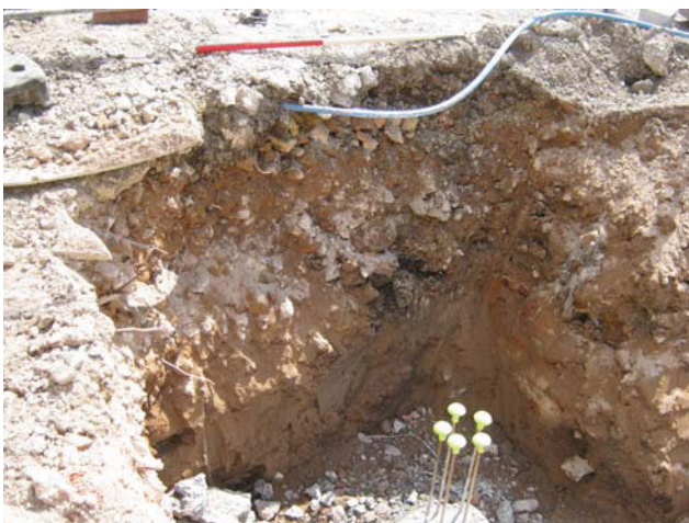
DP 11. W/central foundation trench. Sample section 2. View E.
