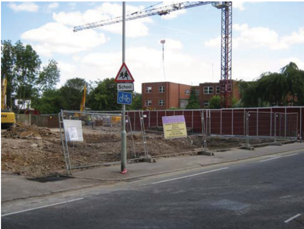
DP 1. 1 High Street, Rickmansworth. View SE.
