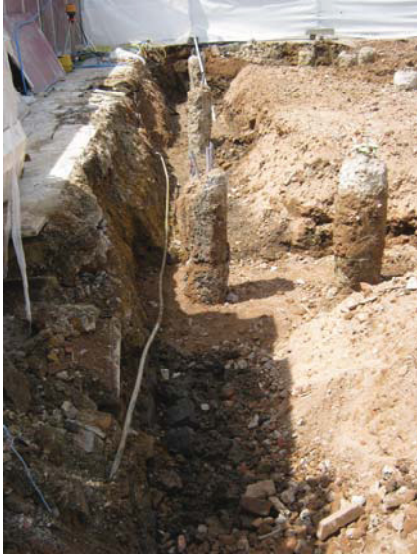
DP 7. S foundation trench. View W.
