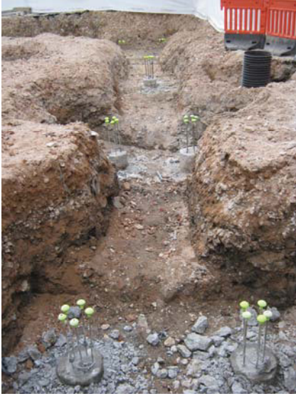
DP 13. N foundation trench. View W.
