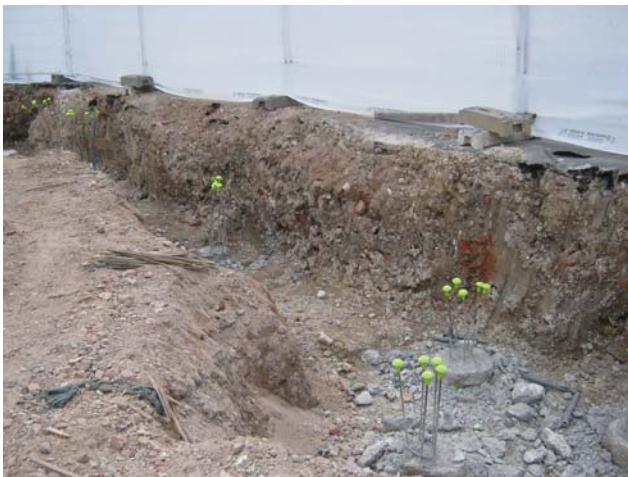
DP 9. W foundation trench. View SW.
