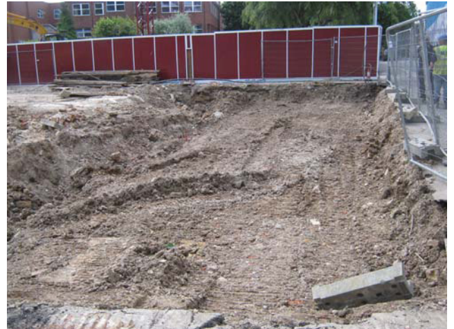
DP 4. W part of the site. View S.
