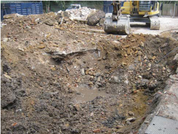
DP 3. Removal of existing paving and foundations. View ENE.
