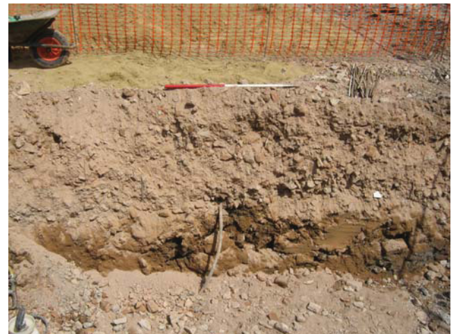
DP 10. S/central foundation trench. Sample section 1. View E.
