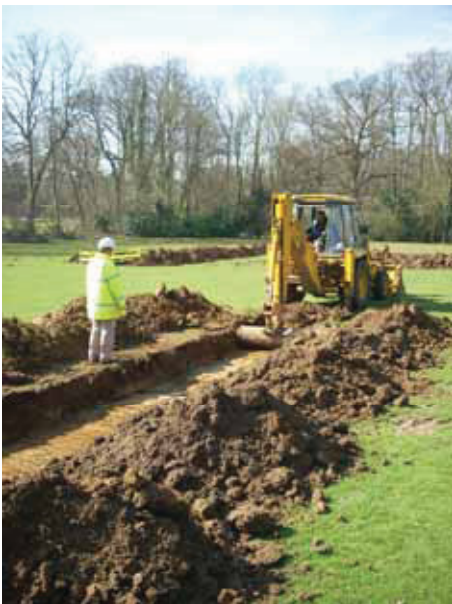
DP 3. Trial trenching. Taken from NE.
