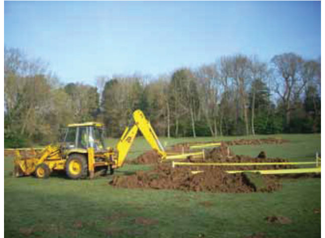
DP 2. Trial trenching. Taken from S.
