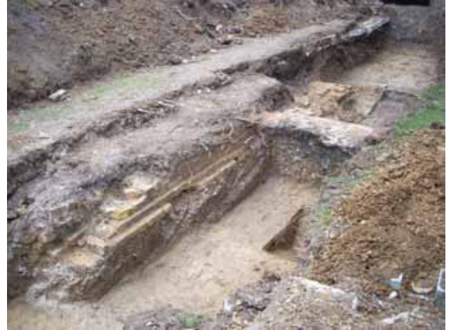
DP 14. Trench 3. Buildings S1029 and S1047 and Ditch F1048. Taken from NE.
