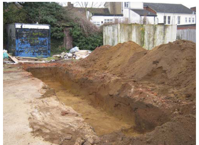
DP 12. Trench 3. View SSE.
