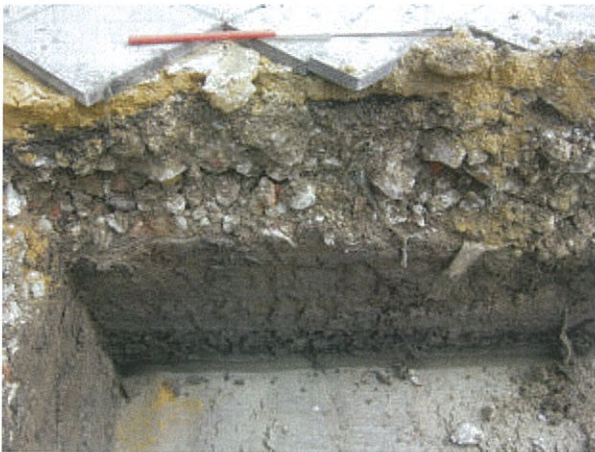
DP 9. Trench 1C, N end. Sample section 1C. View ESE.
