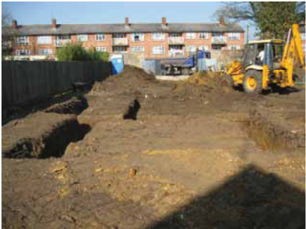
9 General site view. Looking north.
