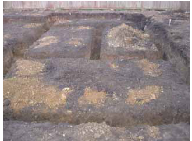
10 Footing trenches. Looking west.
