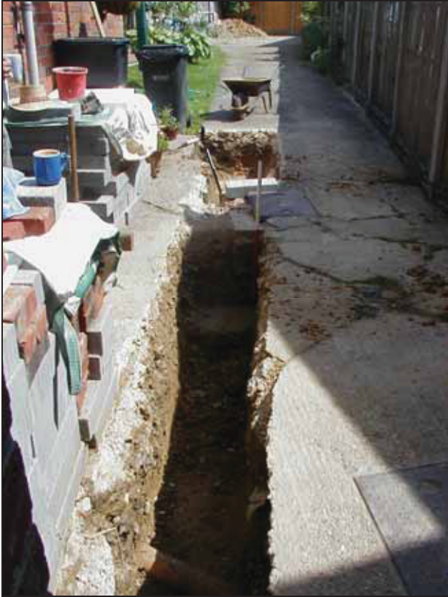
1 Area of excavation. Looking east.
