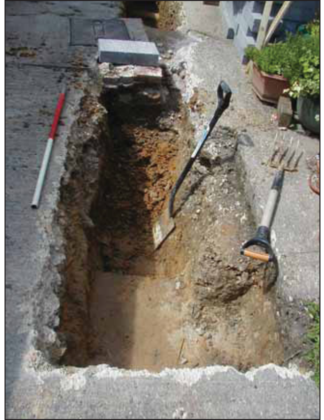
2 Area of excavation. Looking west.
