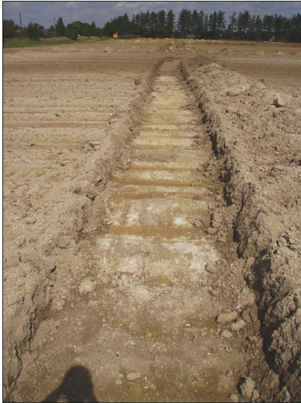
Plate 7 Trial trench 288 looking N
