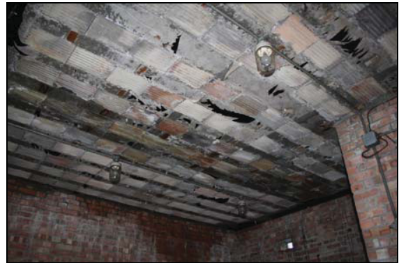
Fire resistant brick roof, Unit 1, interior, Building 13, taken from the south-west
