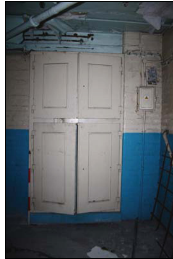
Doors hung on pintles, first floor mezzanine, south side of Building 10, taken from the north-west
