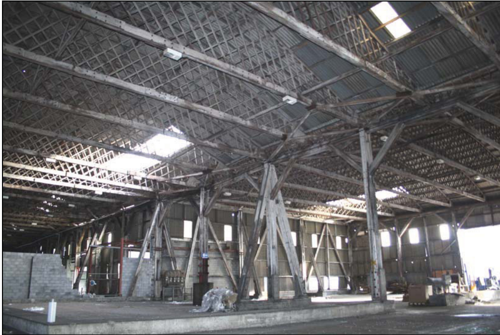
Plate 9 Interior, south-western and south-eastern units, Building 6, taken from the south-west (DP 197)
