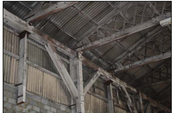
Bracing to the Belfast roof trusses, interior, south-eastern unit, Building 6, taken from the south
