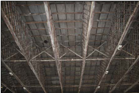
Belfast roof trusses, interior, south-eastern unit, Building 6, taken from the south-west
