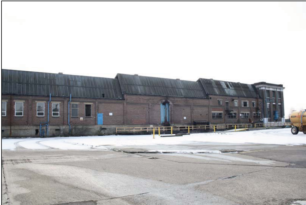
Plate 15 North elevation, Building 10, taken from the north-east (DP 69)
