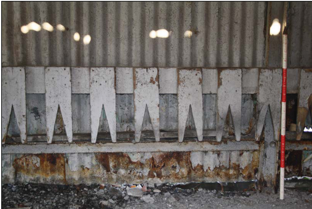
Plate 30 Wooden wall fixings, Building 15, taken from the south (DP 53)
