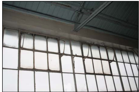
Windows with upper pivoting units, first floor interior, Building 11, taken from the south-west
