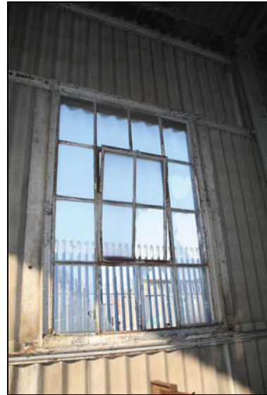
Window with central pivoting section, interior, Building 16, taken from the east
