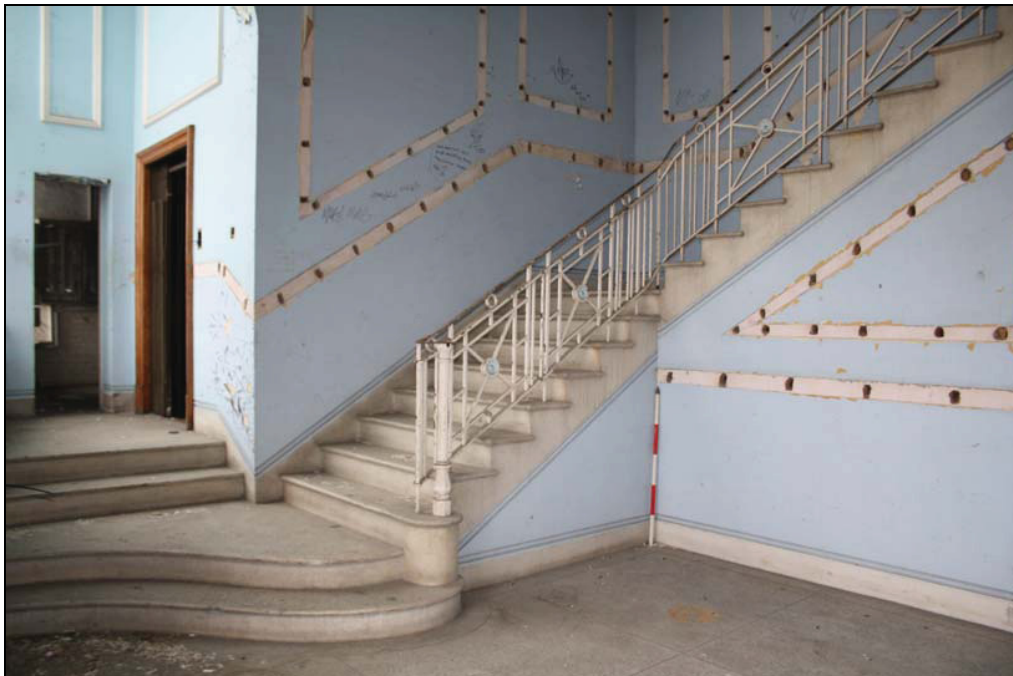
Plate 18 Central staircase, ground floor interior, Building 10, taken from the south-west (DP 138)
