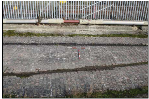
Cobbled surface incorporating narrow gauge train tracks, taken from the south
