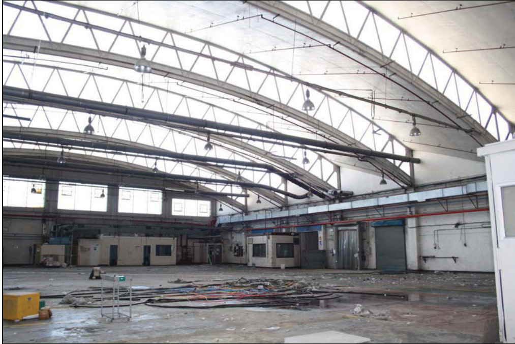
Plate 11 Interior, Building 7, taken from the south-west (DP 204)
