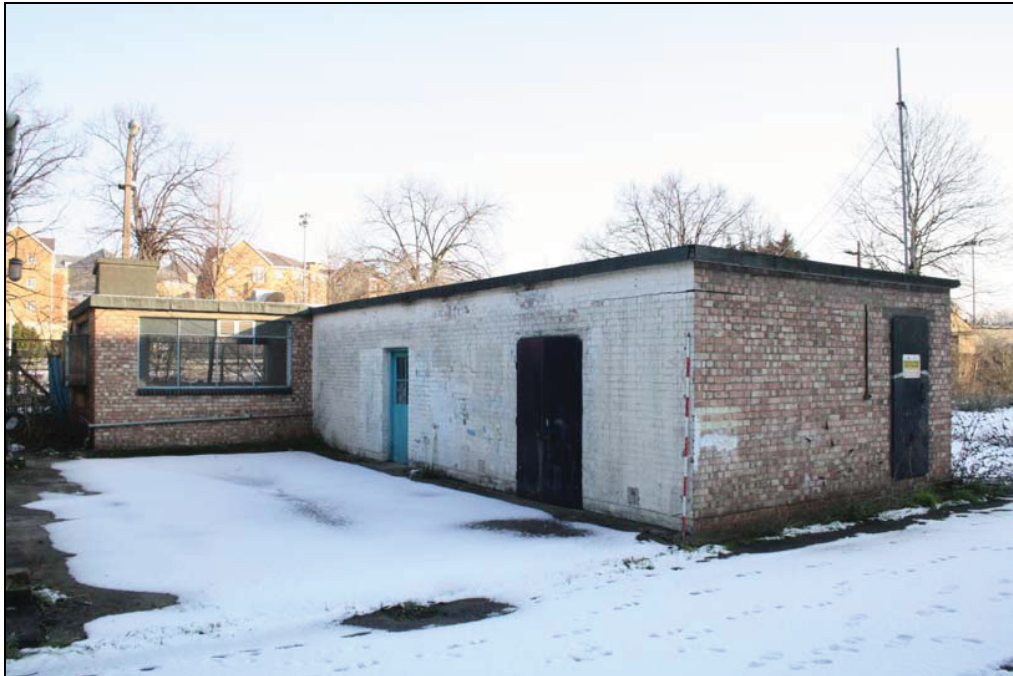
Plate 27 Building 13, taken from the south-west (DP 11)
