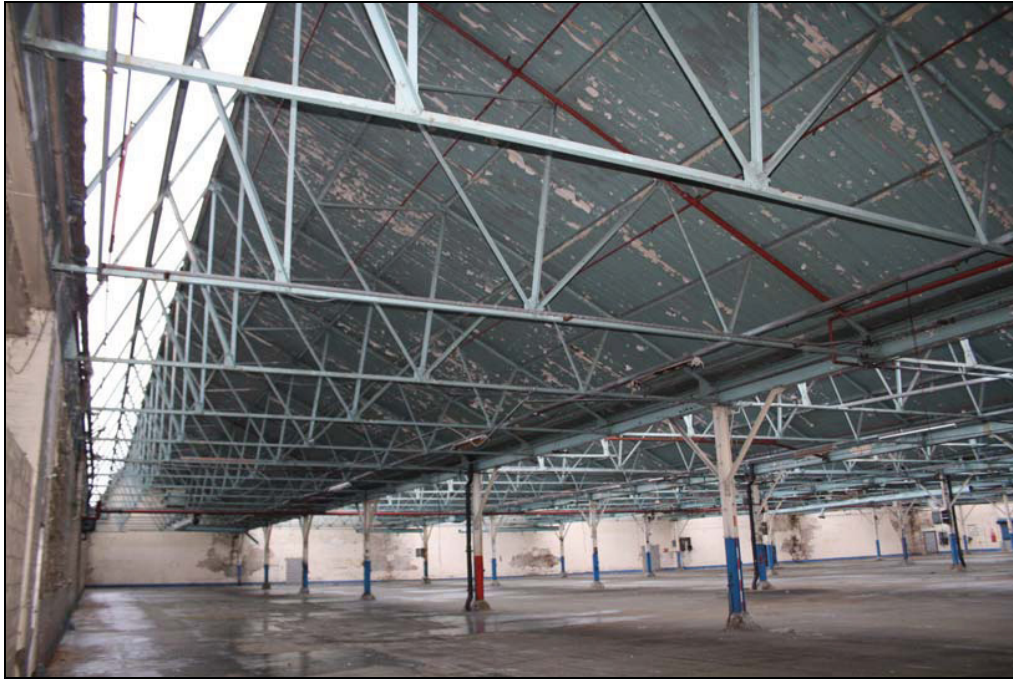
Plate 17 Interior, Building 10, taken from the north-west (DP 98)
