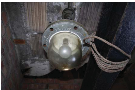
Light with fire resistant glass, Unit 1, interior, Building 13, taken from the south-west
