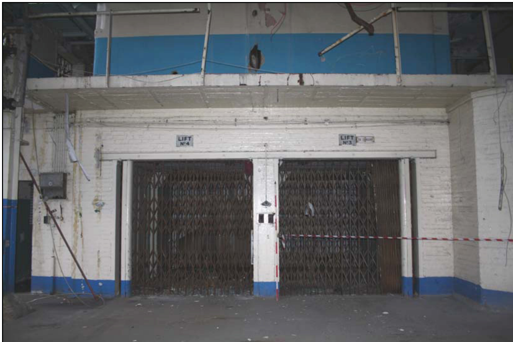
Plate 20 Freight lifts, Building 10, taken from the north (DP 104)
