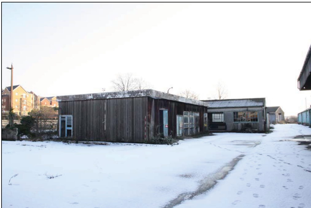
Plate 28 Building 14, taken from the south-west (DP 1)
