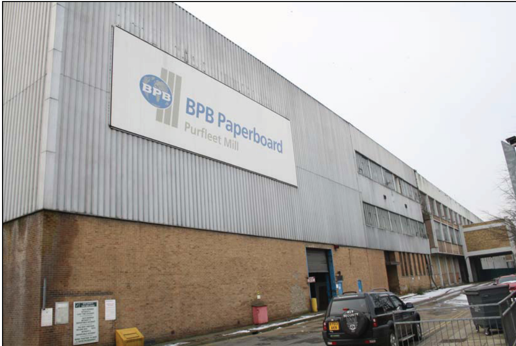
Plate 3 Building 4, north elevation, taken from the north-east (DP 151)
