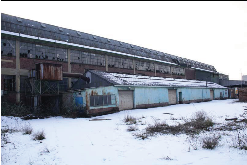
Plate 23 Building 12, taken from the north-east (DP 77)
