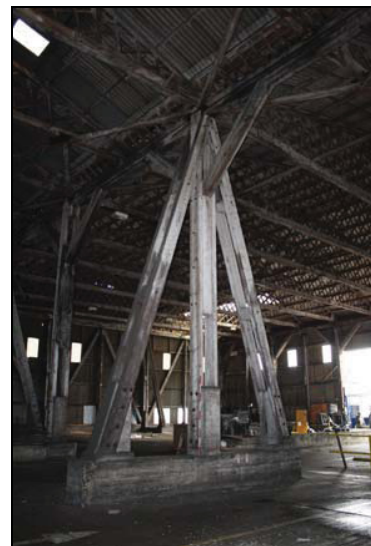
Principal-post supported by long straight braces, interior, south-western and south-eastern units, Building 6, taken from the south-west
