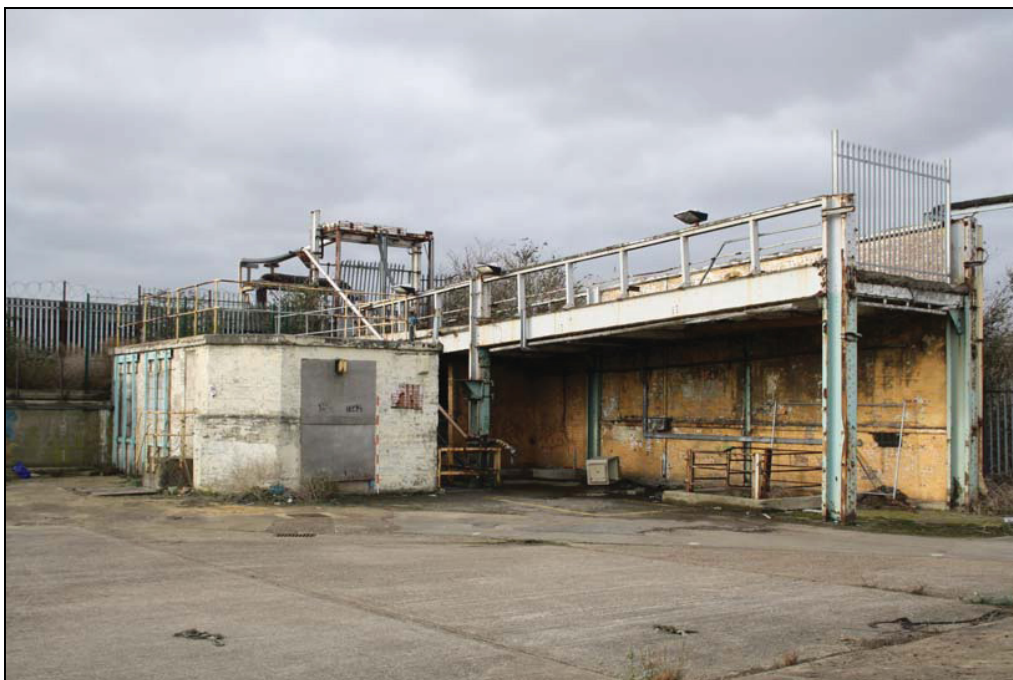
Plate 34 Pump house, Building 19, taken from the north-east (DP 281)
