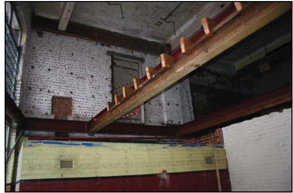
Girders supporting upper floor now removed, Building 10, taken from the south-west
