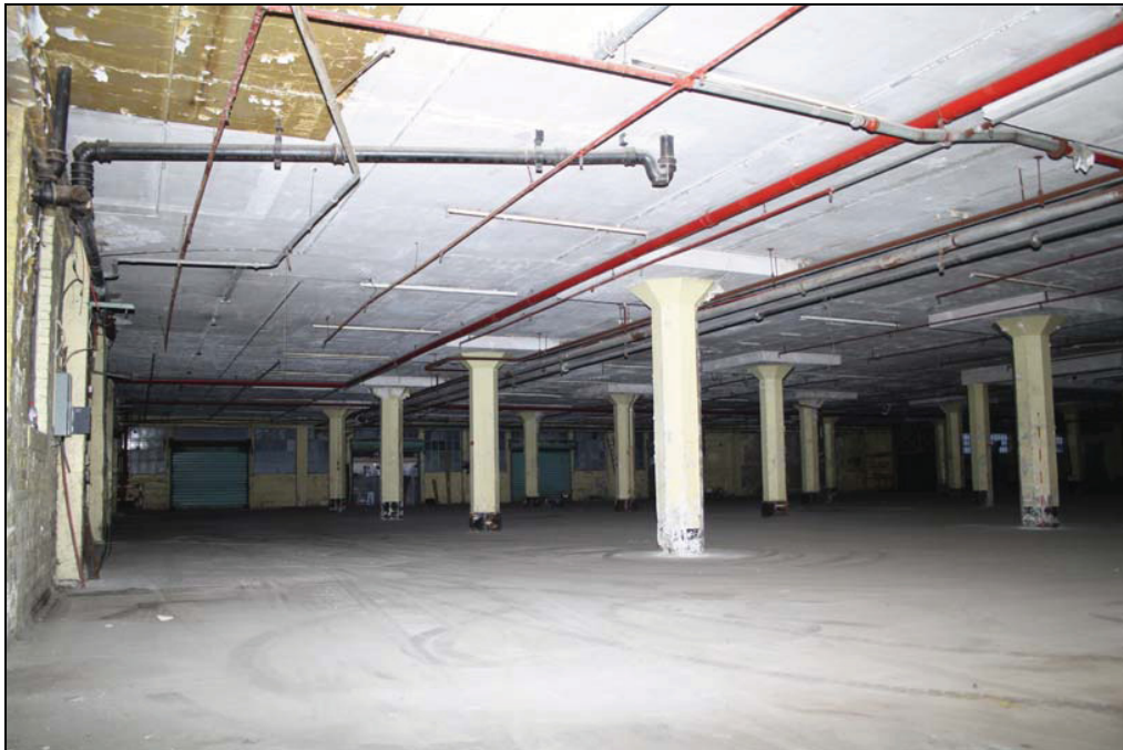
Plate 24 Interior, ground floor, Building 11, taken from the south (DP 85)
