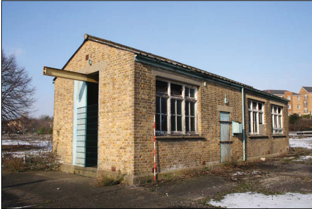
Plate 31 The pump house, Building 17, taken from the south-eastern (DP 55)
