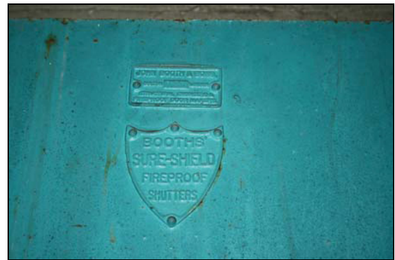
Maker's mark: Booths' sure-shield fireproof shutters, interior, ground floor, Building 12, taken from the north
