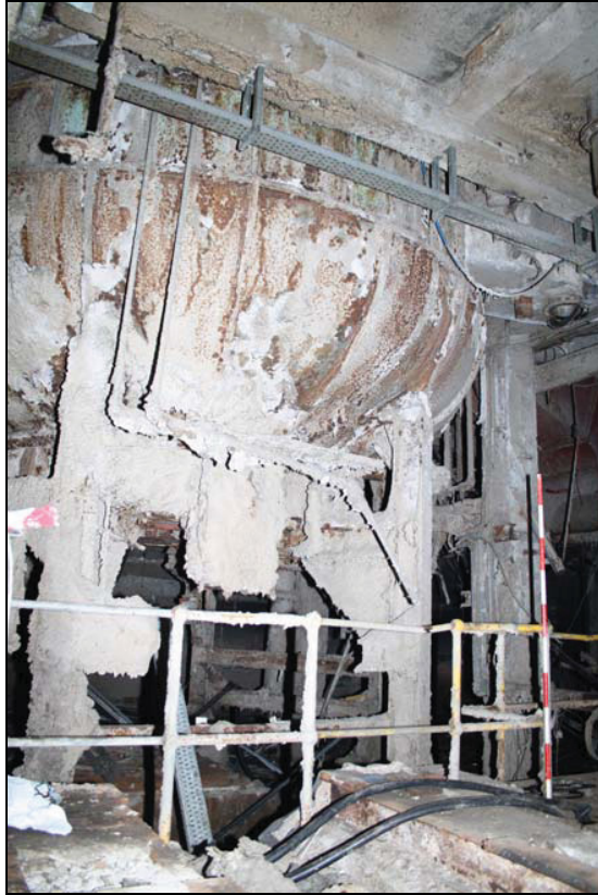
Plate 5 Base of hydro-pulper, ground floor, Building 4, taken from the north-west (DP 217)
