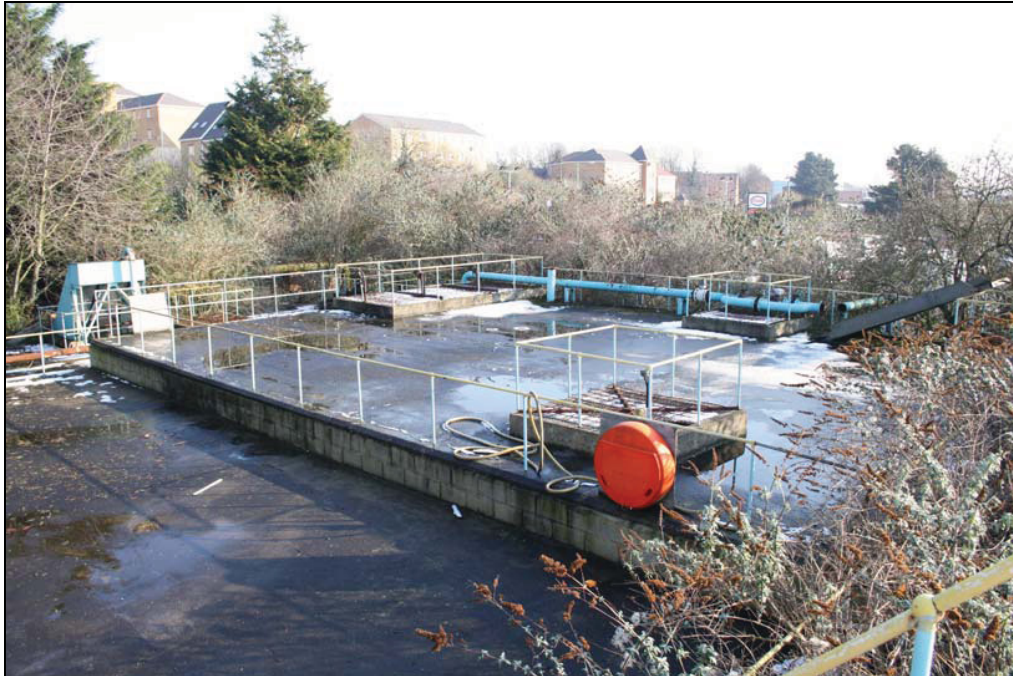
Plate 33 Reservoir, Building 18, taken from the south-east (DP 33)
