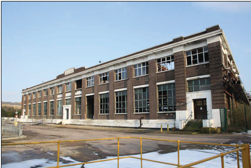
Plate 13 Main frontage, west elevation, Building 10, taken from the south-west (DP 84)
