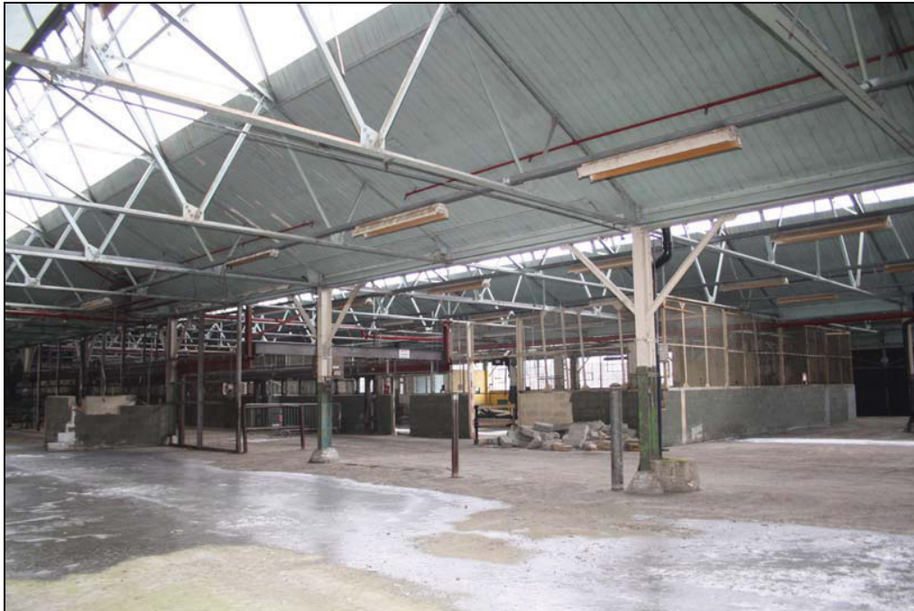
Plate 25 First floor interior, Building 11, taken from the south-east (DP 126)
