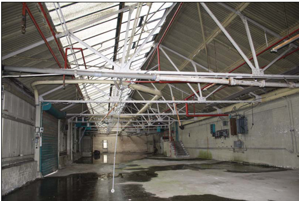
Plate 26 Open warehouse, interior, Building 12, taken from the west (DP 143)
