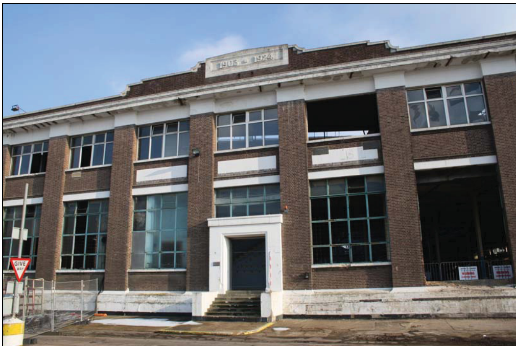
Plate 14 Main frontage, west elevation, Building 10, taken from the west (DP 82)
