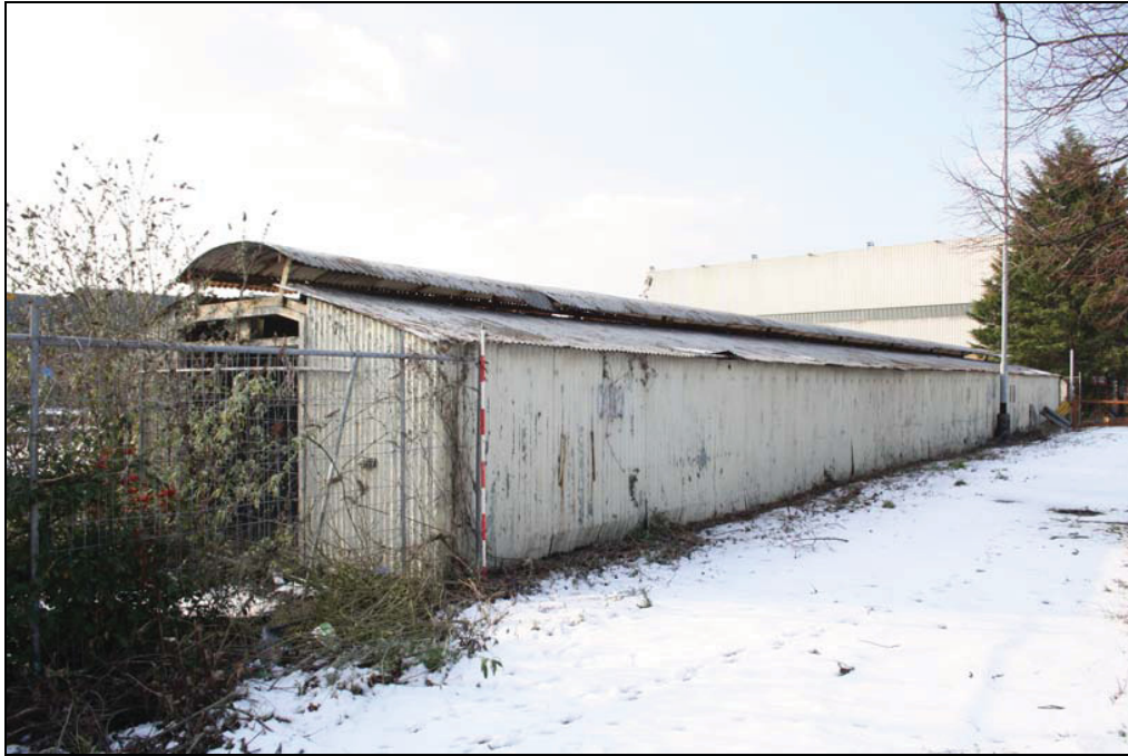
Plate 29 Building 15, taken from the north-east (DP 47)
