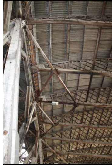
Bracing to the Belfast roof trusses, interior, south-eastern unit, Building 6, taken from the south
