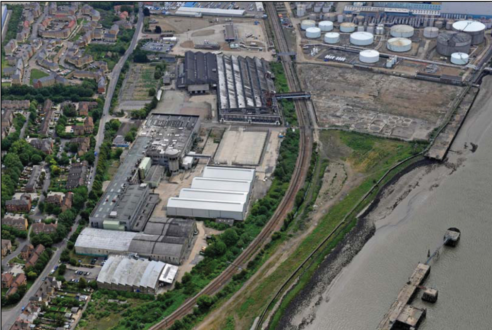
Plate 2 Aerial view of BPB Paperboard, Purfleet, taken from the west
