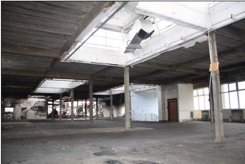
Plate 22 Second floor interior, Building 10, taken from the north-east (DP 134)
