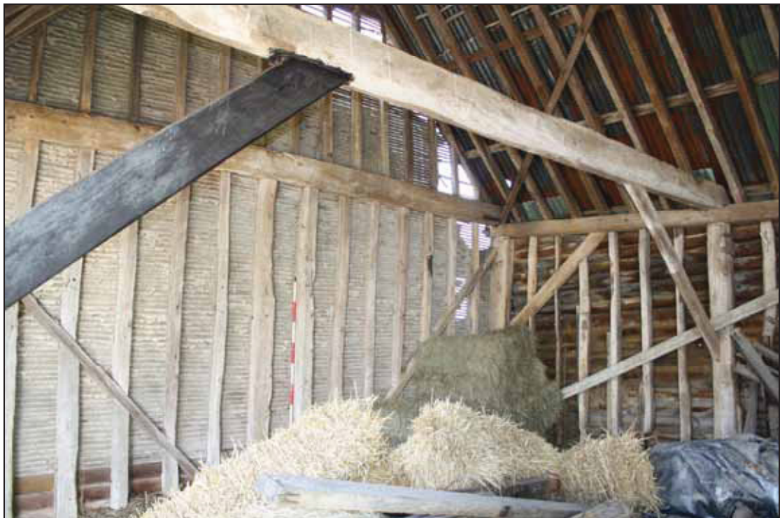
Plate 12 South wall of Building 2, taken from the north-east (DP 31)
