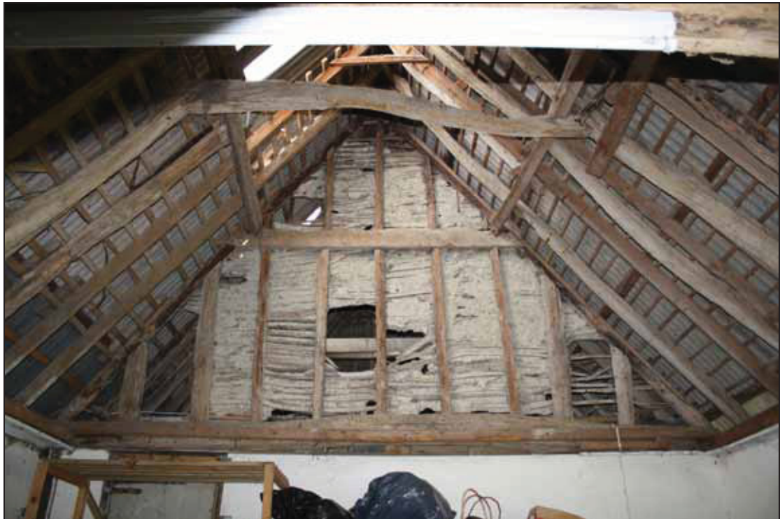
Plate 15 Studwork partition between Bays 5 and 6 (Building 3), taken from the south (DP 27)
