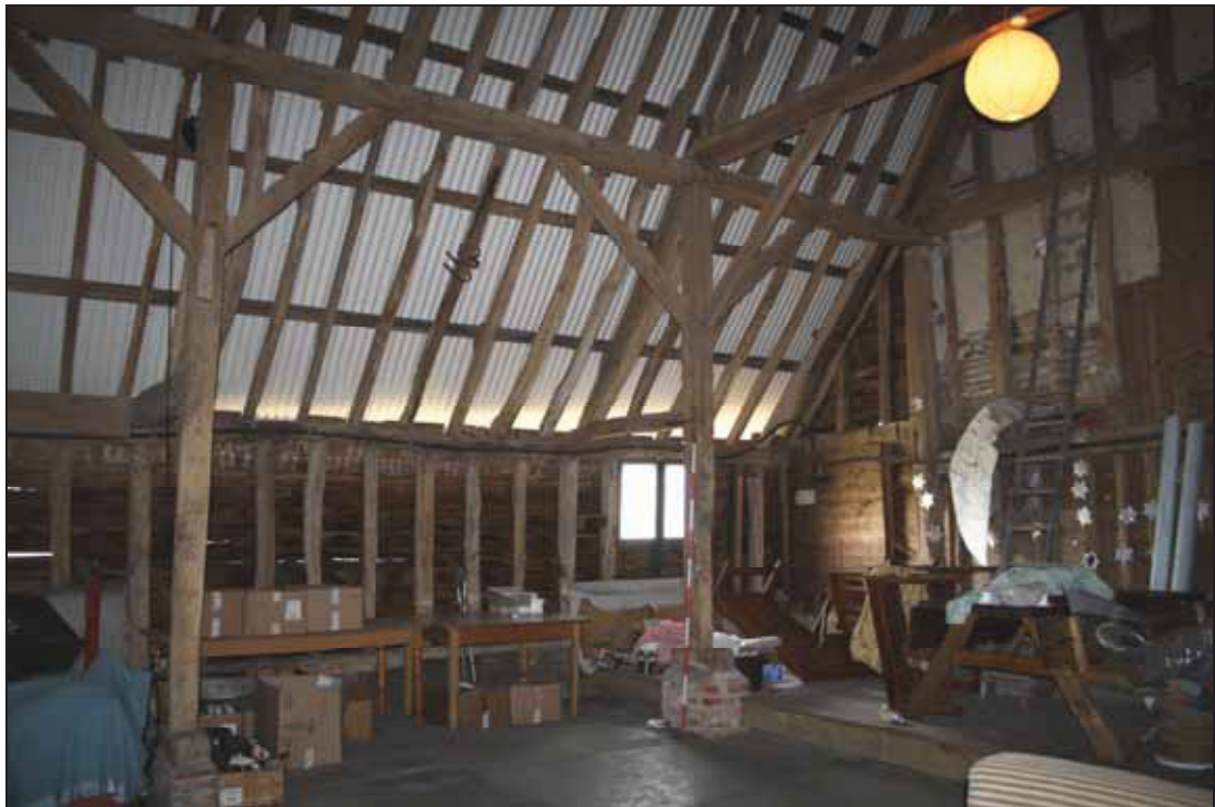
Plate 4 West side of Bays 1 and 2, taken from the south-east (DP 42)
