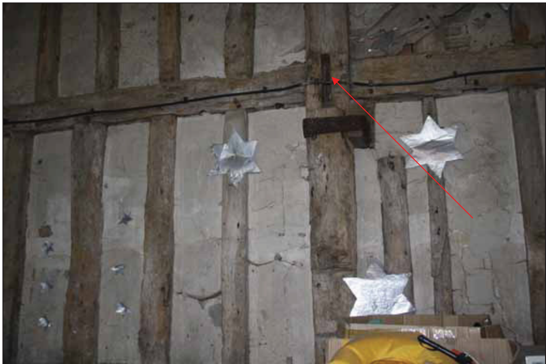
Plate 6 East side of Truss 4 (Building 1) showing original window position in Bay 4 and mortise for lateral binding joist (indicated), taken from the west (DP 53)
