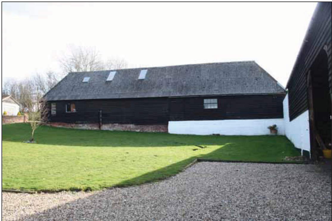
Plate 14 West elevation of Building 3, taken from the west (DP 03)
