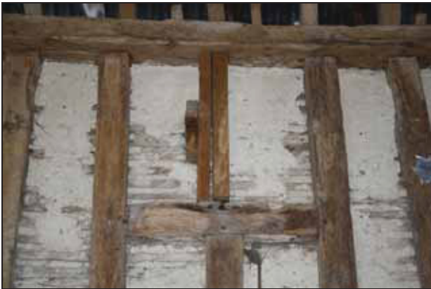
DP 45 Original upper window on the east side of Bay 2 (Building 1), taken from the west
