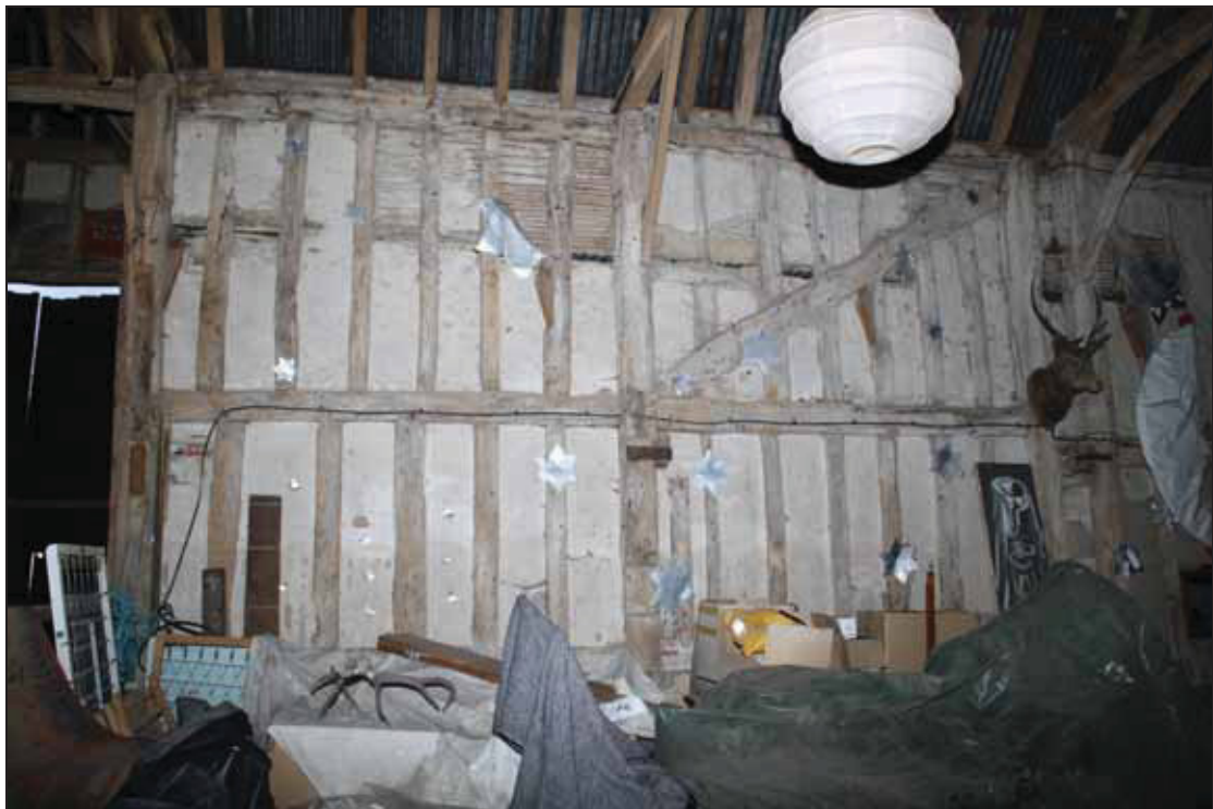
Plate 2 East side of Bays 4 and 5, taken from the west (DP 48)
