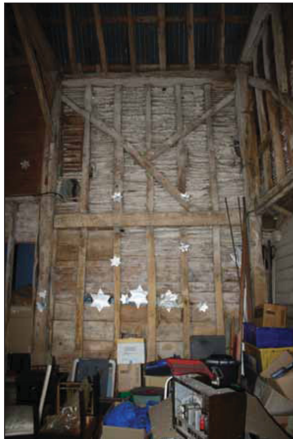
Plate 10 East side of Bay 8, taken from the west (DP 61)
