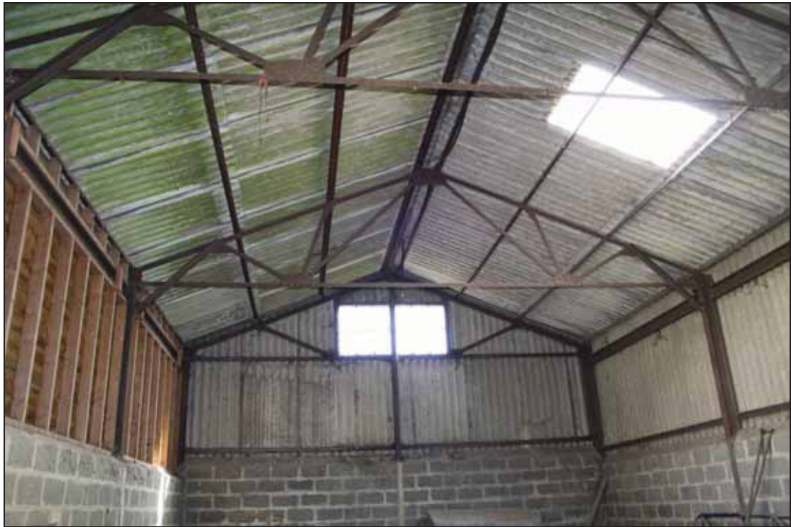
Plate 17 Roof structure of Building 4, taken from the west (DP 23)
