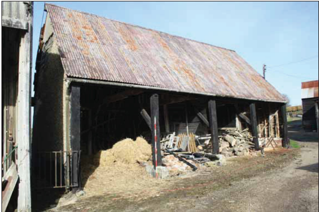
Plate 11 East elevation of Building 2, taken from the south-east (DP 01)
