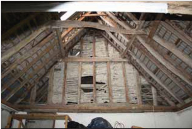
DP 27 Studwork partition between Bays 5 and 6 (Building 3), taken from the south
