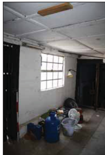
DP 66 East side of Unit 1 (Building 1), taken from the north-west
