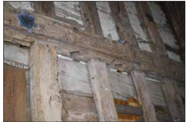
DP 46 Position of original lower window on the east side of Bay 2 (Building 1), taken from the north-west
