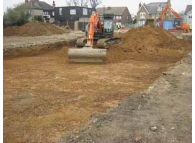
2 General view of the basement excavations. Looking north west.
