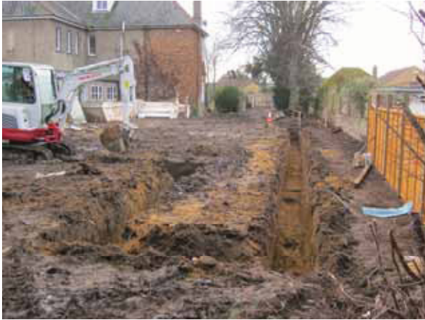
19 Mid-excavation view of garage footings. Looking south.
