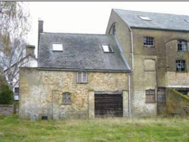
DP 7: View of Bowman's Mill taken from the west with Mill House behind. The area in the foreground is proposed to contain a new building
