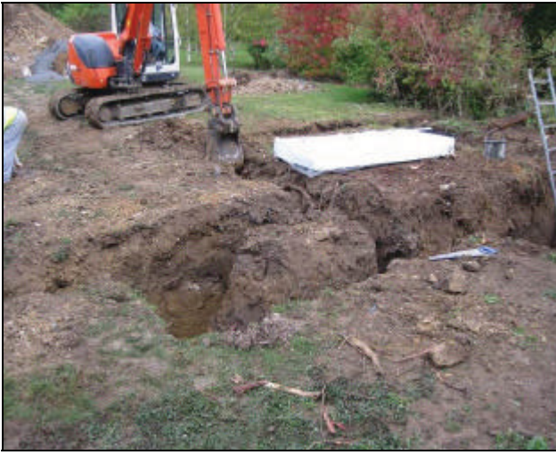
DP.7 Mid excavation. Looking north.
