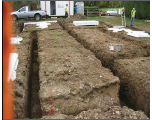
DP.8 Post excavation. Looking south.
