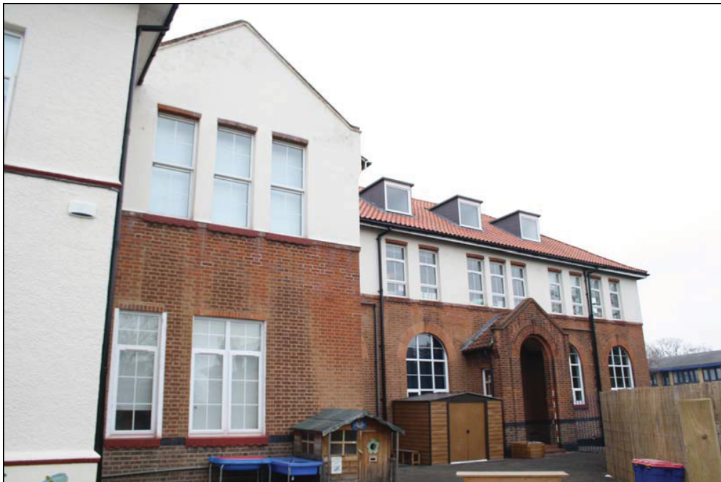
Plate 4 1940s eastern extension, south elevation, taken from the south-west (DP 4)
