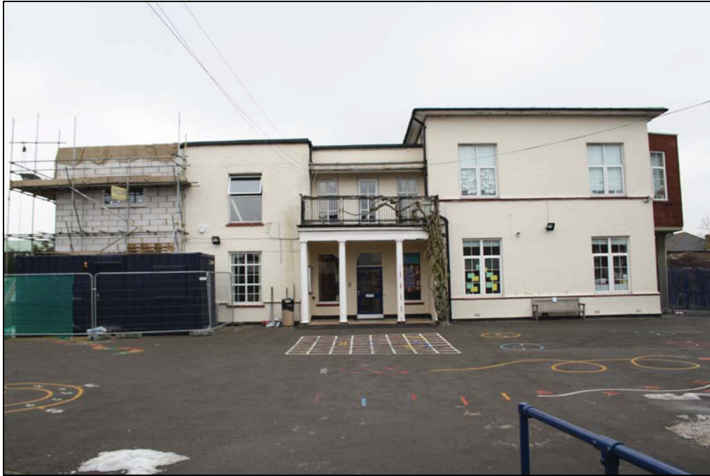
Plate 3 Original entrance and new extension, west elevation, taken from the west (DP 6)
