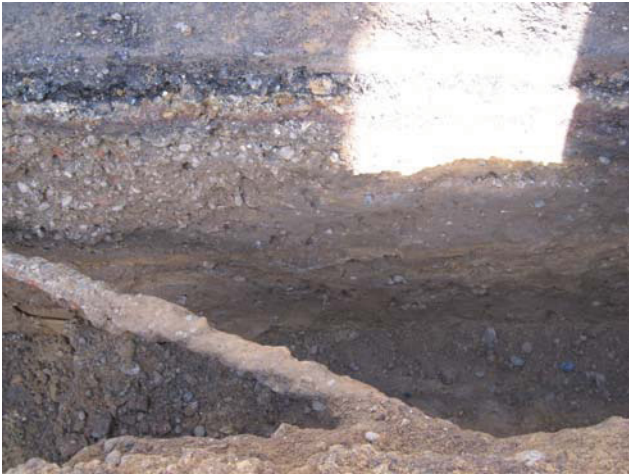
DP 3. North foundation trench. Sample section 1. Looking north-north-west.
