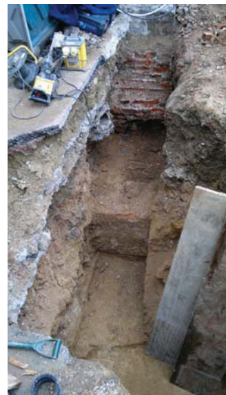
DP 6. South-western foundation/service trench. Looking west.
