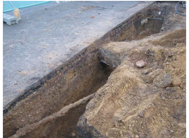
DP 2. North foundation trench. Looking north-east.
