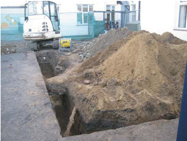
DP 1. The site. Foundation trenches. Looking east.
