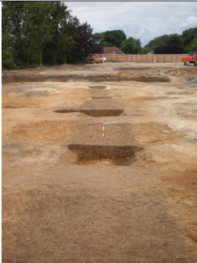
6: Enclosure Ditch F2159 (and earlier Ditches F2161 and F2163 beneath), view N
