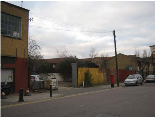
DP 1. 123 Fairfield Road, Bow. Looking north-west.
