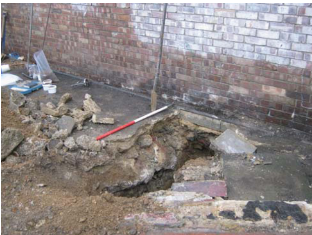
DP 5. Test Pit 2A. Looking south-south-east.
