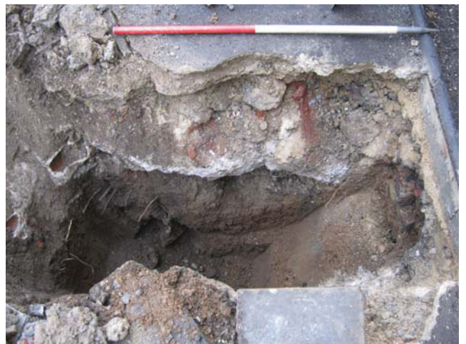
DP 6. Test Pit 2A. Eastern section. Looking north-east.
