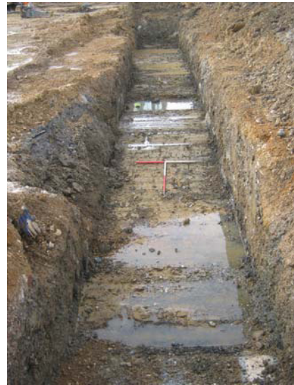
DP 10. Trench 3. Looking west.
