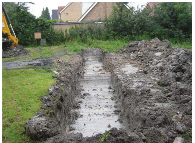
DP 6. Trench 2. Looking north-west.
