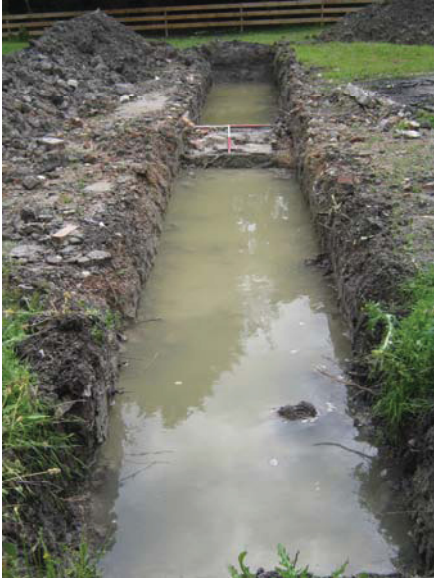
DP 7. Trench 2. Looking south-east.
