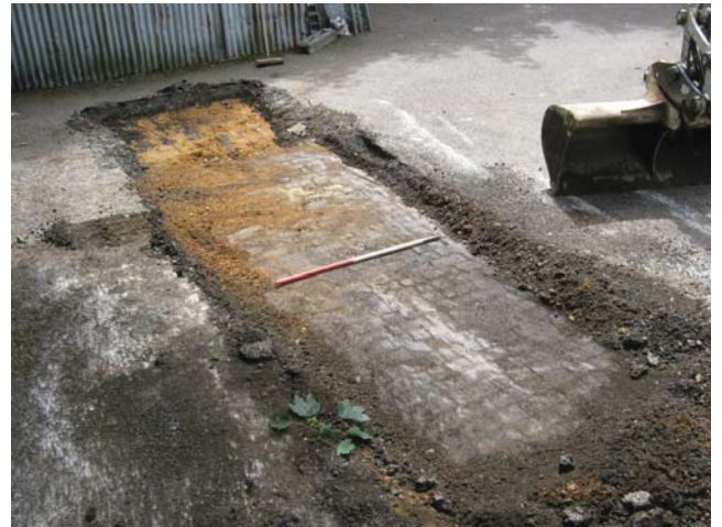
DP 2. Trench 1 during excavation. Floor/yard surface M1014. Looking south.
