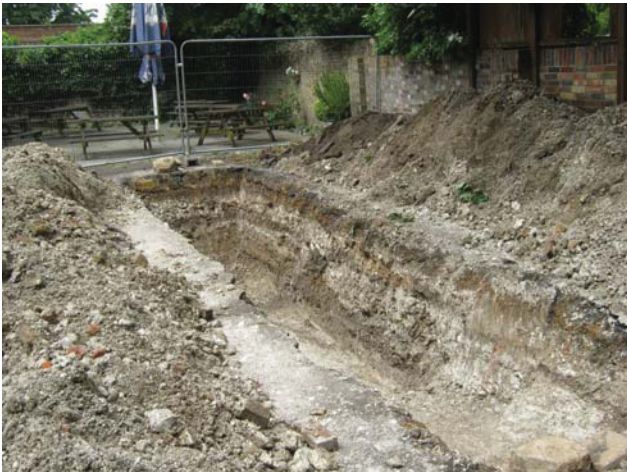
DP 9. Trench 1, general view. Looking north.
