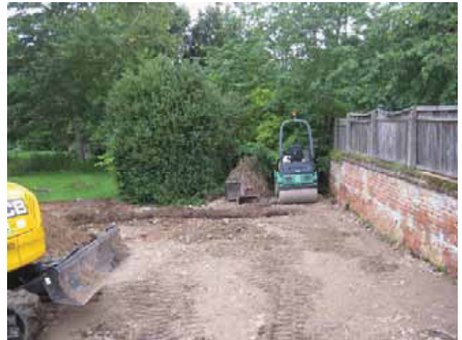
DP 2. Northern part of the site. Looking north-north-west.
