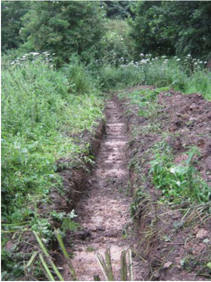
DP 1. Trench 1. Looking south-south-west.
