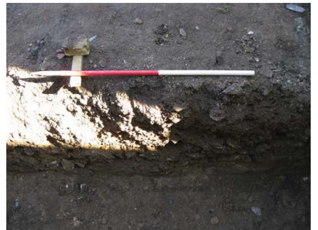
DP 4. Trench for a new retaining wall. Sample section 1. Looking east-south-east.
