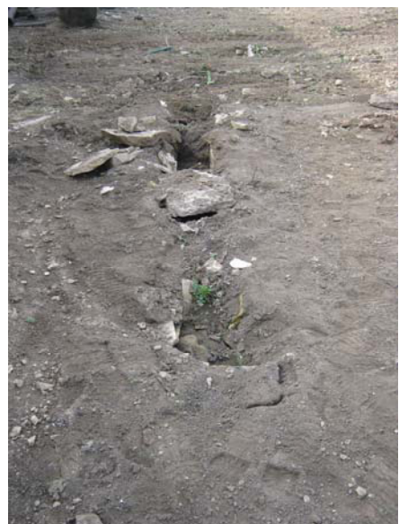
DP 12. Remains of a culvert. Looking south-west.
