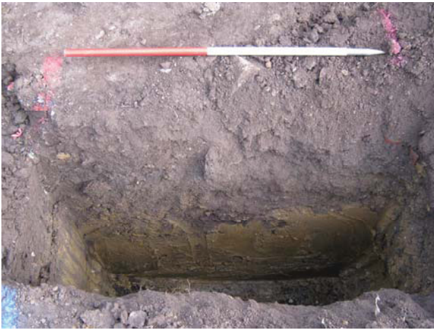
DP 7. North-western part of foundation trench. Sample section 4. Looking north-north-east.
