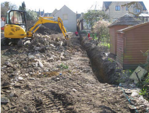
DP 3. Trench for a new retaining wall. Looking south-south-west.
