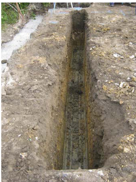
DP 11. Western part of foundation trench. Looking north-north-east.
