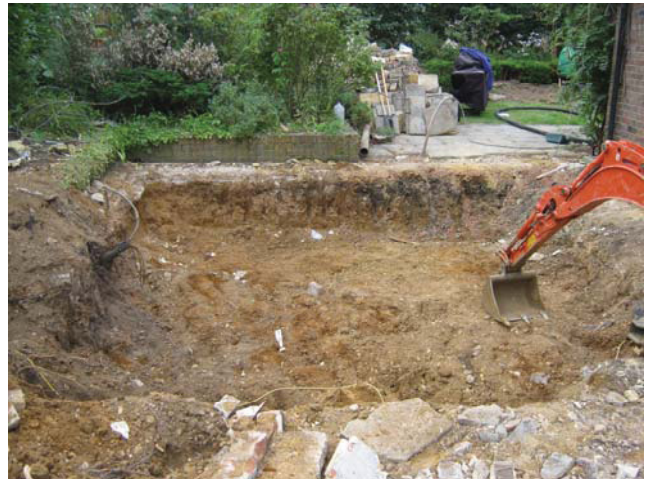
DP 2. The southern part of the excavation. Looking south.
