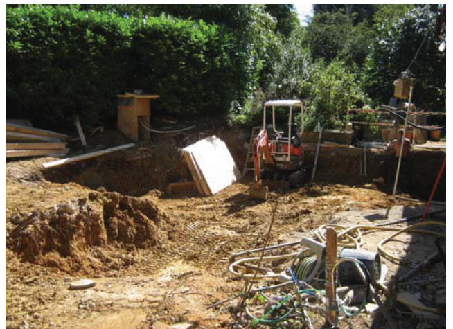
DP 6. The excavation area. Looking south-east.
