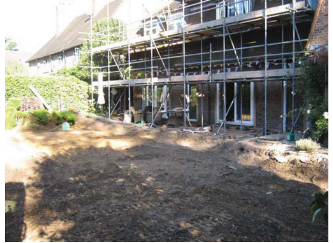
DP 8. Rear of the house. Looking north-west.
