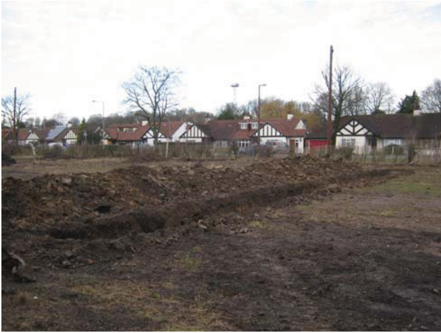
DP 1. Trench 1. Looking north-west.
