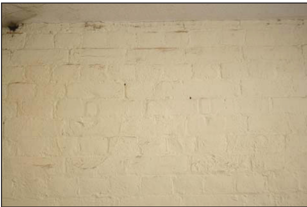
Impressions for former pattress plates on the west wall of Room GF10 (Building 1), taken from the east
