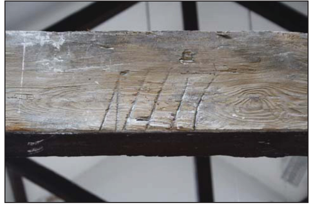
Bracking mark on a tie-beam of the roof over Building 1, taken from the west
