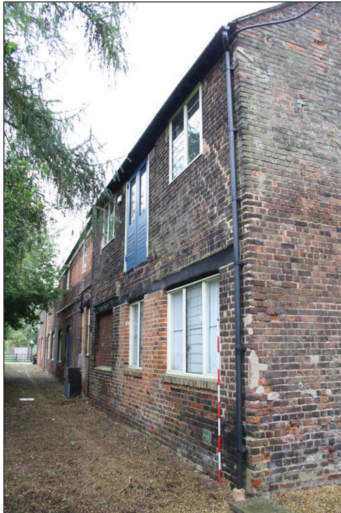
12 East elevation of Building 2, taken from the north-east (DP 20)
