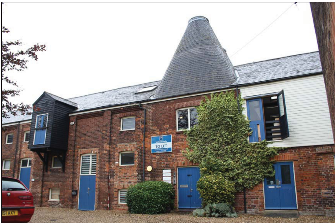
2 South elevation of Building 1 showing kiln cone, taken from the south-east (DP 07)
