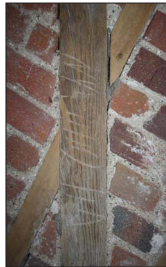
Baltic bracking mark on a primary brace on south side of Room MF01 (Building 1), taken from the north
