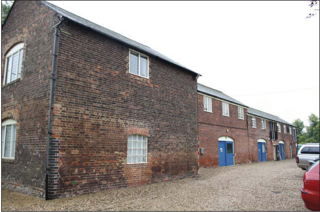
11 West elevation of Building 2, taken from the north-west (DP 12)
