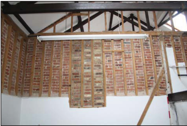
Blocked aperture in the partition between the steeping bays and the germination floors at upper level (Building 1), taken from the west
