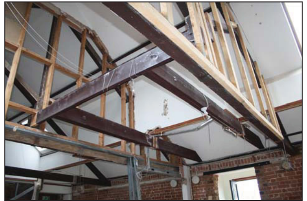
Later timber framework supporting the floor on the south side at upper level (Building 1), taken from the north-west
