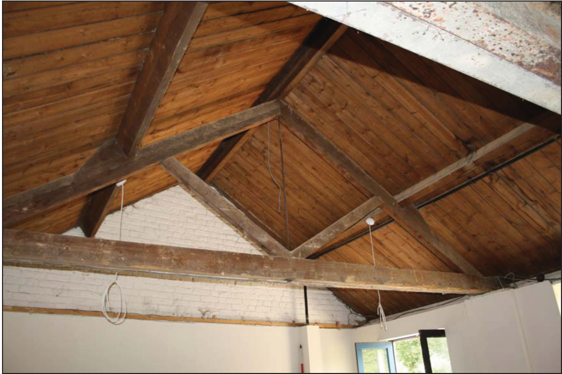
13 Roof truss over Room FF02 (Building 2), taken from the north (DP 61)
