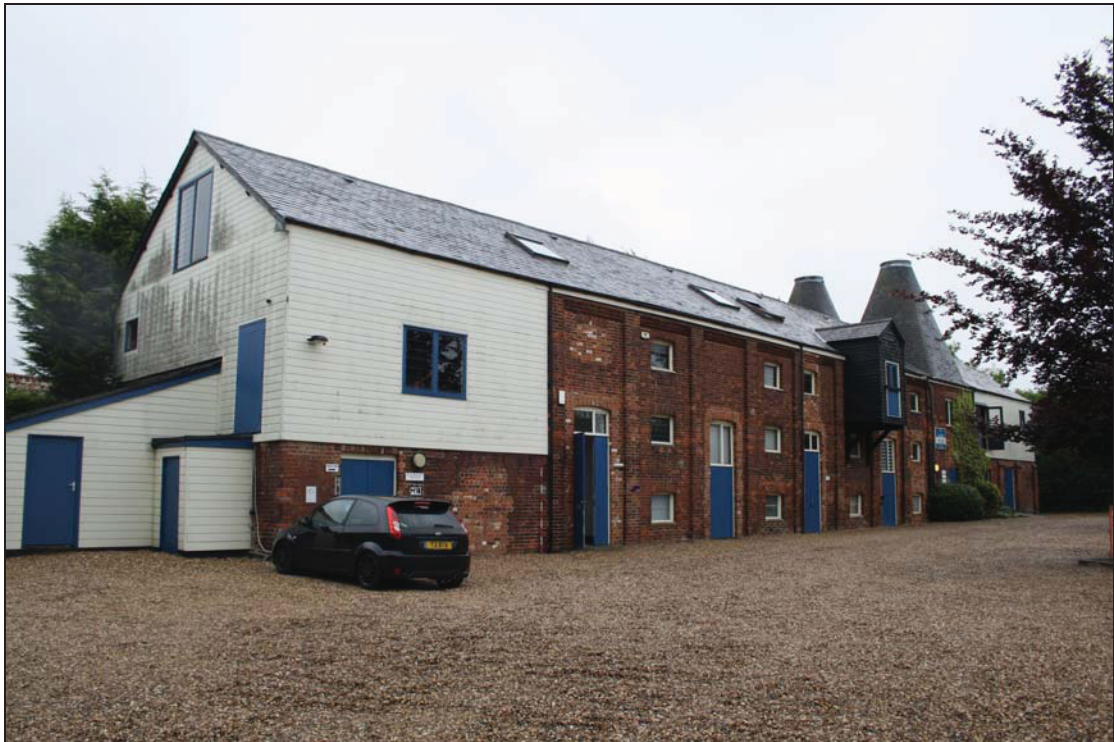
1 South elevation of Building 1, taken from the south-west (DP 04)
