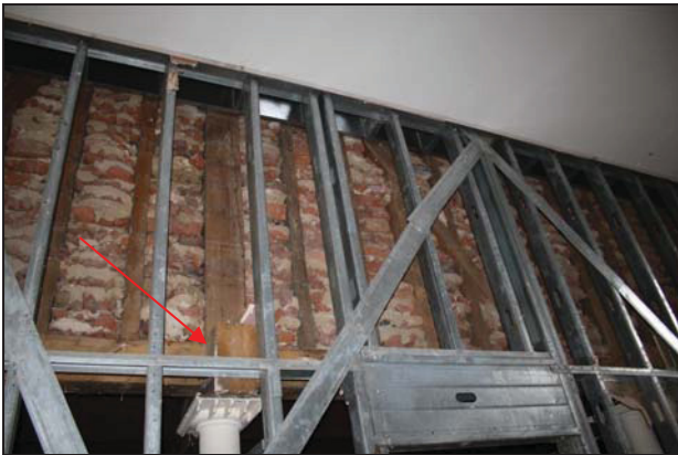
Detail of the junction between the steeping bays and malting floor showing truncated bridging joist (indicated) (Building 1), taken from the east
