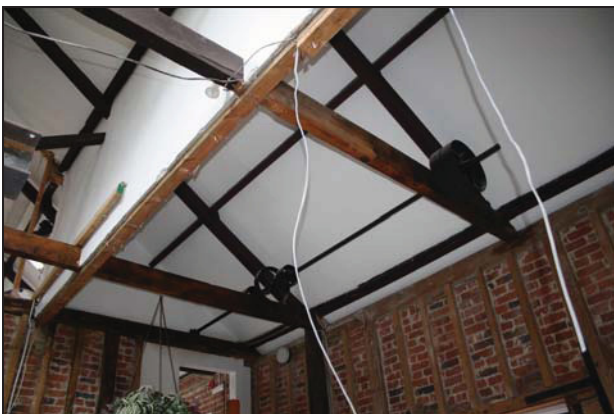
View of roof over the steeping bays showing a driveshaft (Building 1), taken from the north-west
