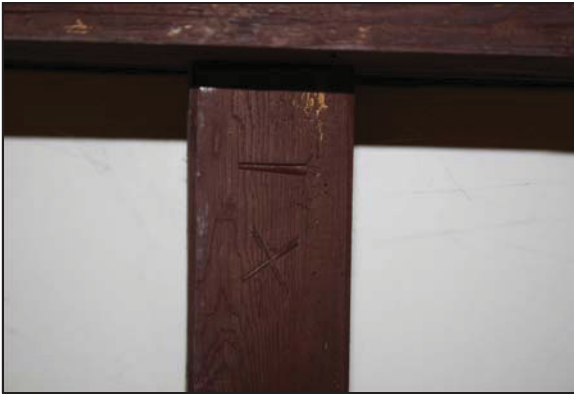
Assembly mark on an original ceiling joist in Room GF03 (Building 1), taken from the north
