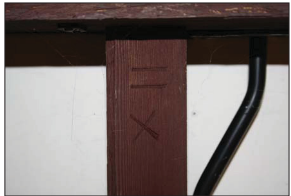
Assembly mark on an original ceiling joist in Room GF03 (Building 1), taken from the north
