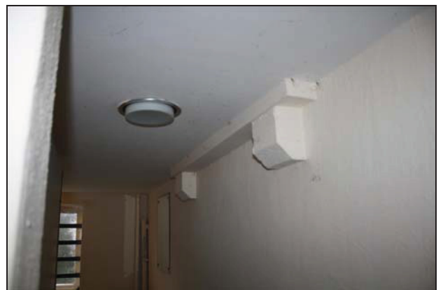
Infilled apertures (indicated) for metal tie-rods to support the former drying floor of the kilns (Building 1), taken from the south
