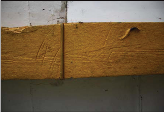
Baltic bracking mark on the principal ceiling joist in Building 3, taken from the east
