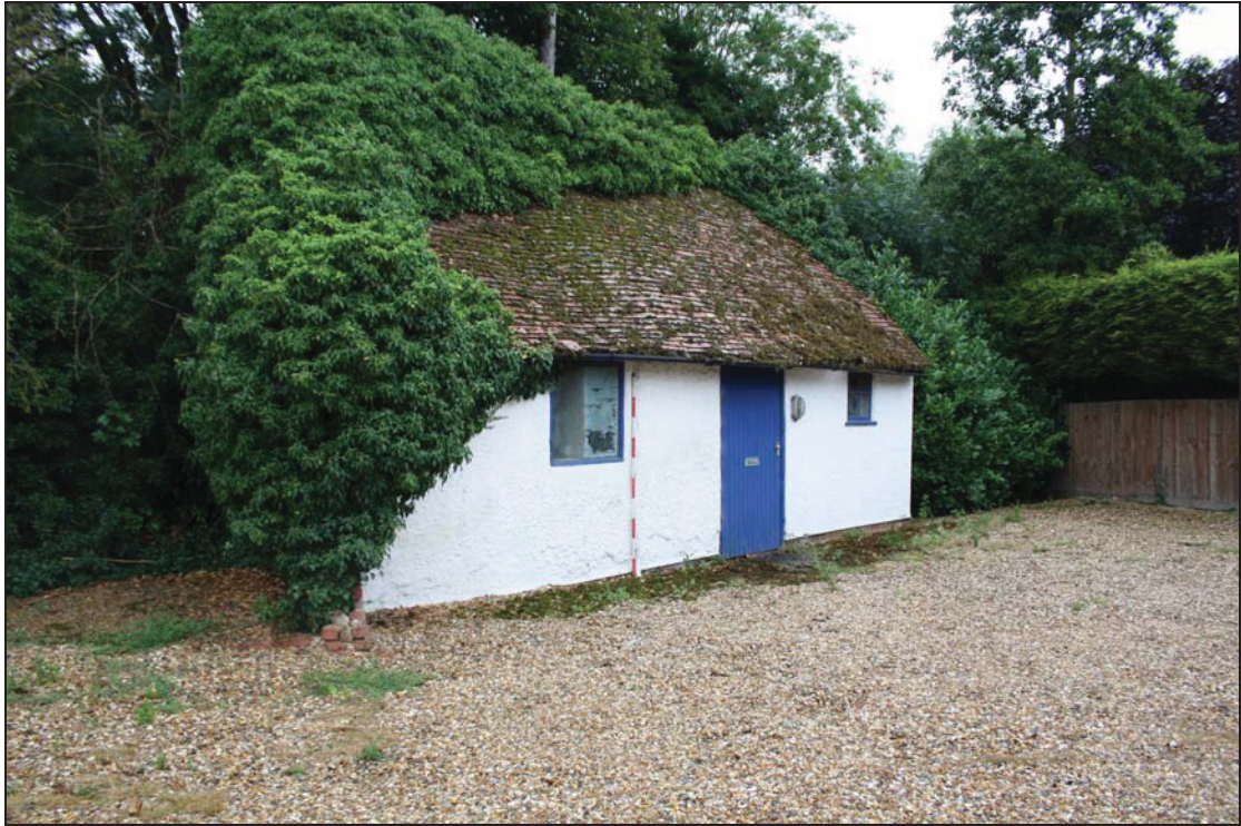
15 Building 3, taken from the south-east (DP 01)
