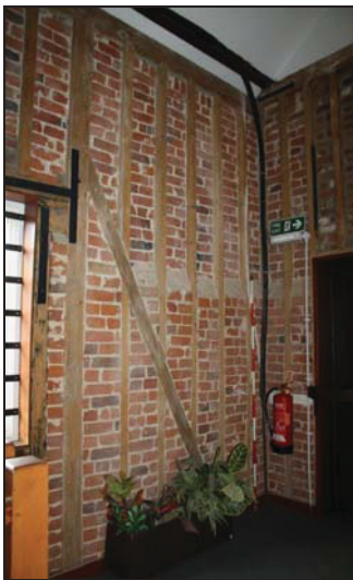
Primary braced studwork on the south side of the staircase in Room GF01 (Building 1), taken from the north
