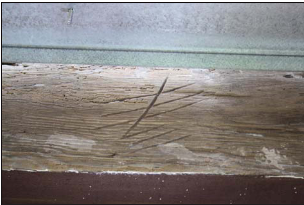
Bracking mark on a tie-beam of the roof over Building 1, taken from the west
