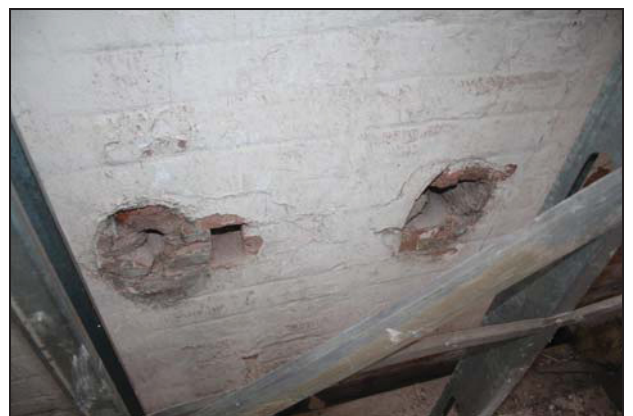
Evidence for pattress plates for tie-rods to the kilns (Building 1), taken from the west
