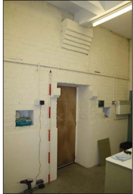
West side of Room GF10 showing doorway into north kiln and corbelling for the joist above (Building 1), taken from the south-east
