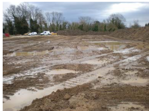
DP 6. General Shot – East view
