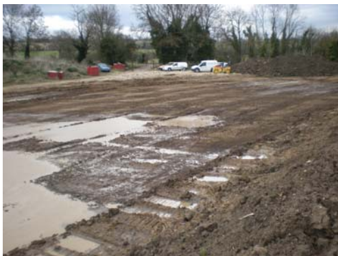
DP 5. General Shot – North East view
