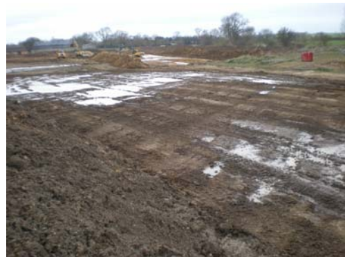
DP 4. General Shot – North West view
