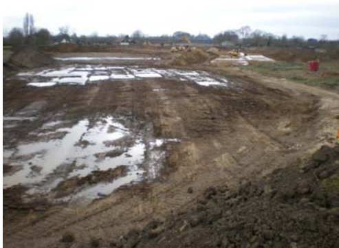
DP 3. General Shot – West view
