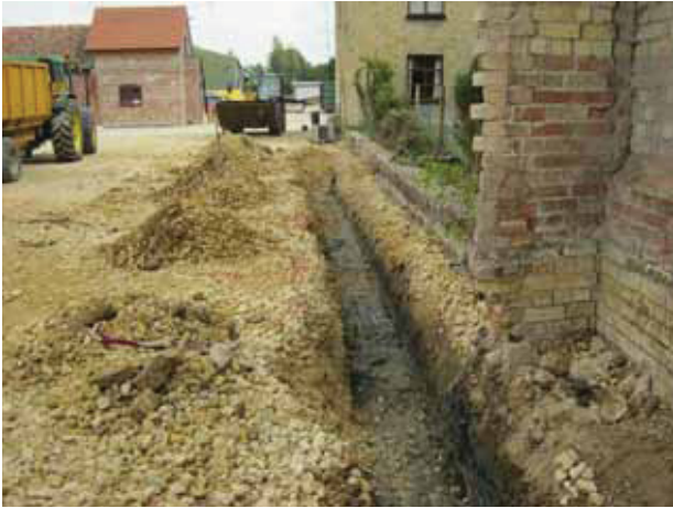
7 General view of footings along south east edge. Looking north east.
