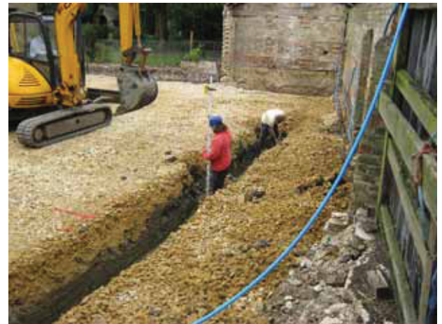
4 General view of footings in western corner. Looking east.
