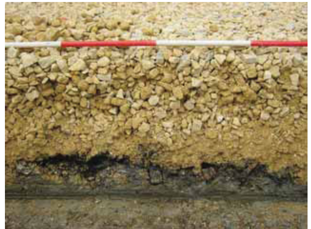
10 Sample section 4. Looking north west.
