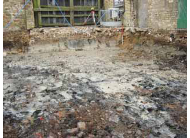
2 L1002 exposed in western corner. Looking south west.
