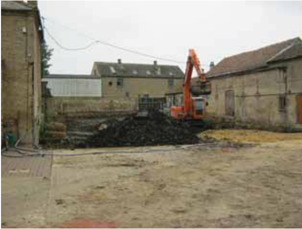
1 General view during later stages of demolition work. Looking south west.
