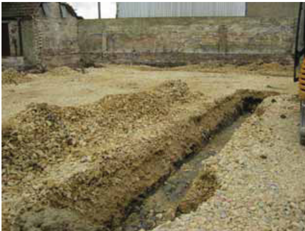
9 General view of central footings. Looking south.
