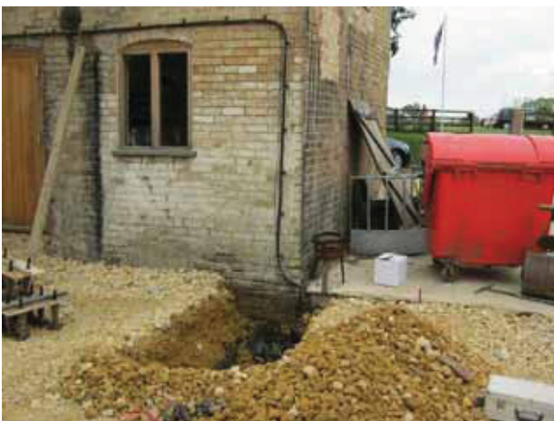
11 General view of footings in northern corner. Looking north west.
