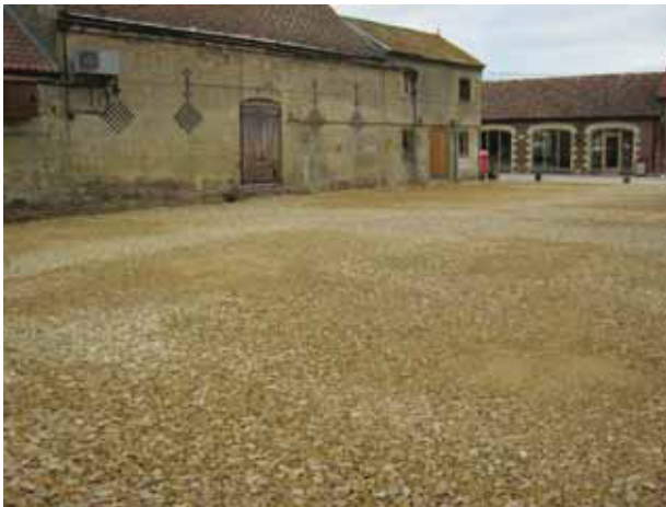
3 General view after reinstatement of ground level. Looking north.
