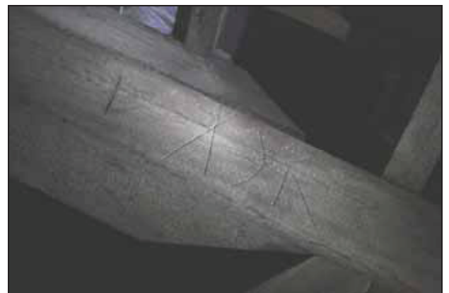
Baltic batch mark on a principal rafter in the roof (Anne Knight Building), taken from the south
