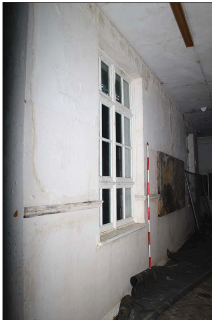
20 Ground floor west corridor (Law Building), taken from the north-west (39)
