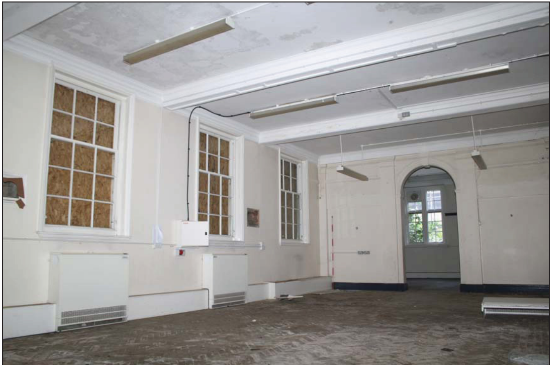
9 Room GF07 (Frederick Chancellor Building), taken from the west (89)
