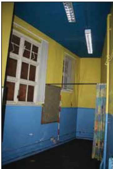
41 Room GF09 (Law Building), taken from the south
