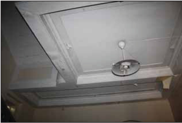
Entrance hall GF01 (Law Building), taken from the north
