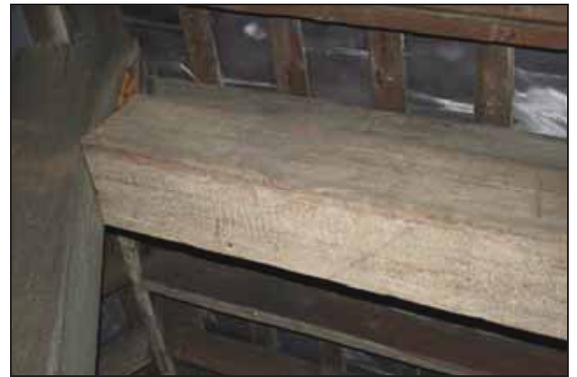
Baltic batch mark on a principal rafter in the roof (Anne Knight Building), taken from the south
