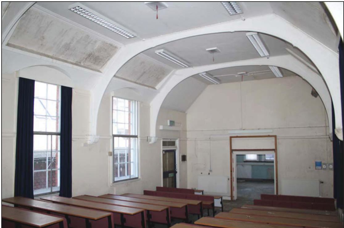
14 Room FF10 (Frederick Chancellor Building), taken from the south-west (104)
