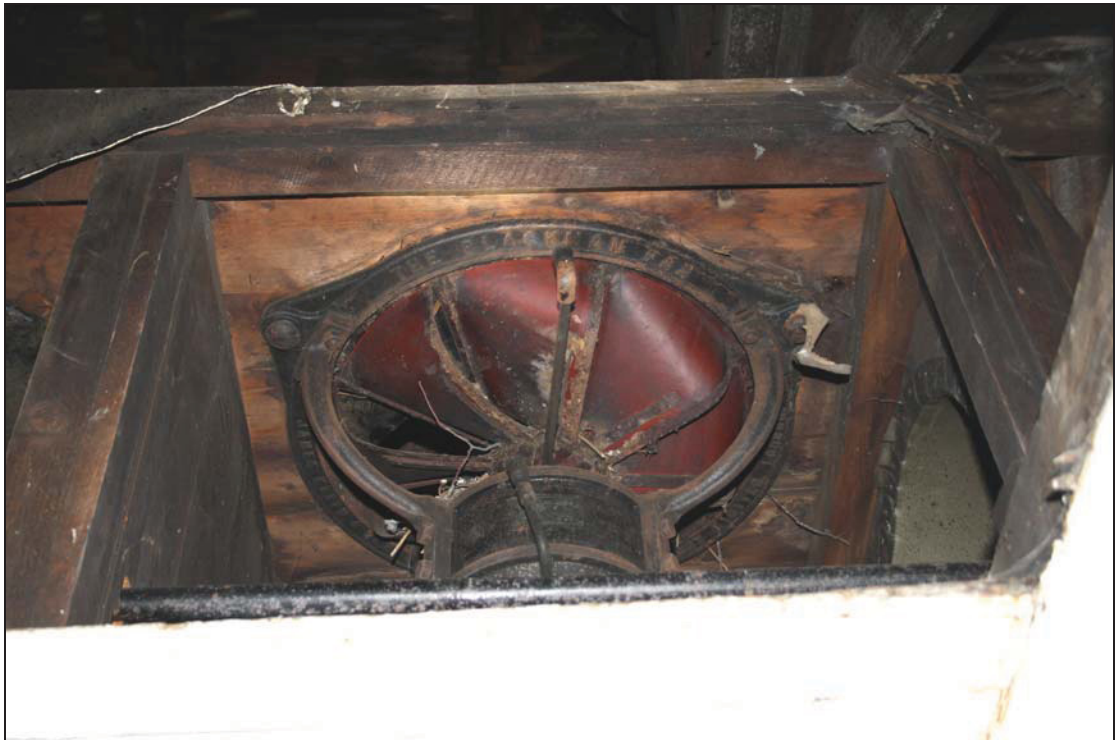
15 North-west side of Room SF05, taken from the south-east (65)
