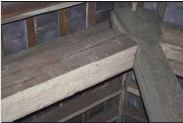
Baltic batch mark on a principal rafter in the roof (Anne Knight Building), taken from the south
