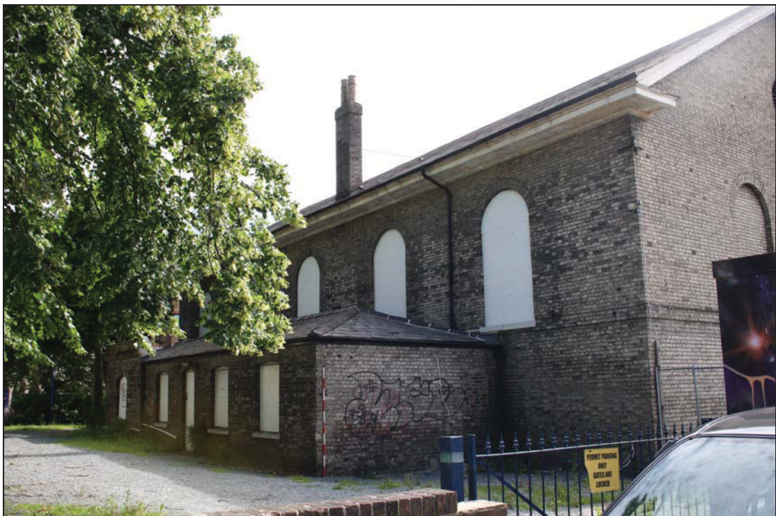
2 West elevation, taken from the south-west (01)
