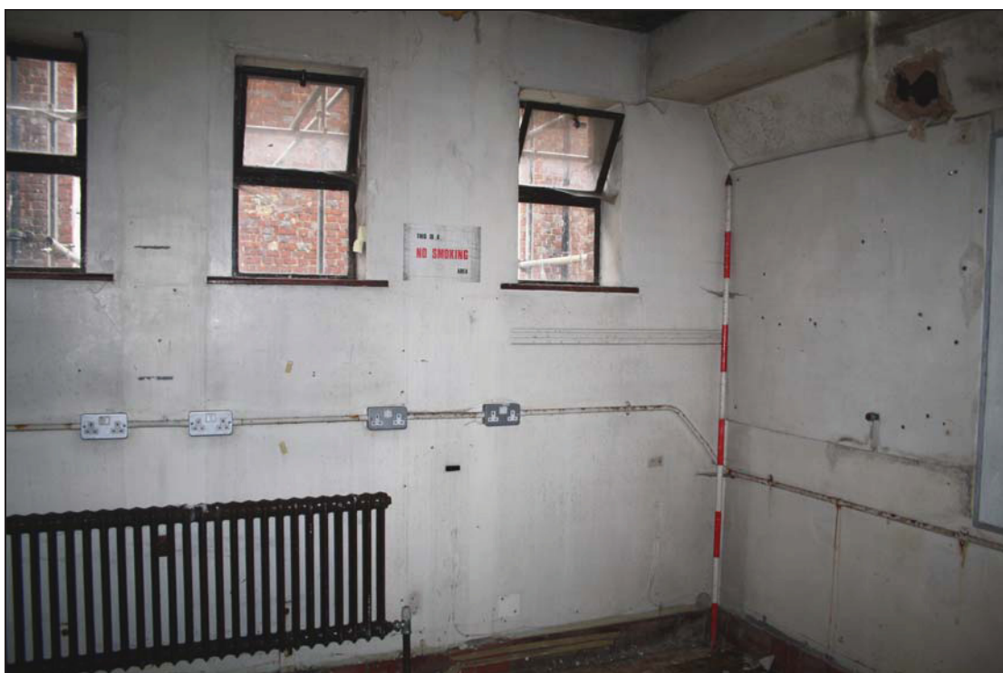
11 Room FF02c (Frederick Chancellor Building), taken from the south-east (99)
