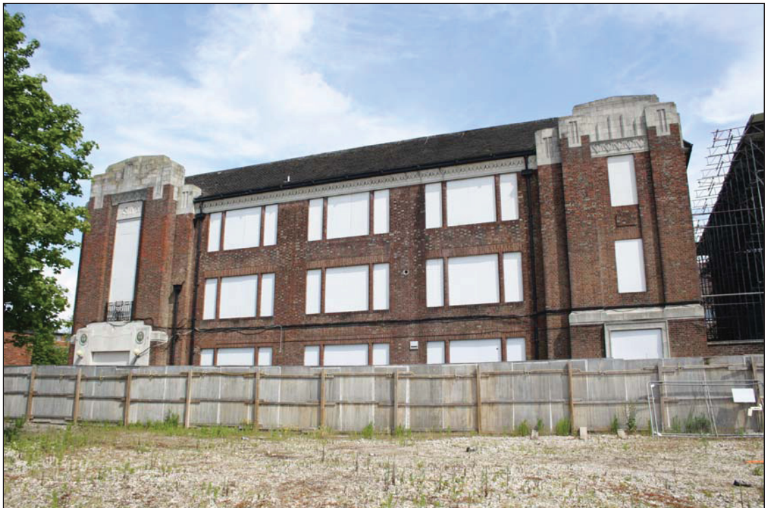
16 South elevation of the Law Building, taken from the south (11)
