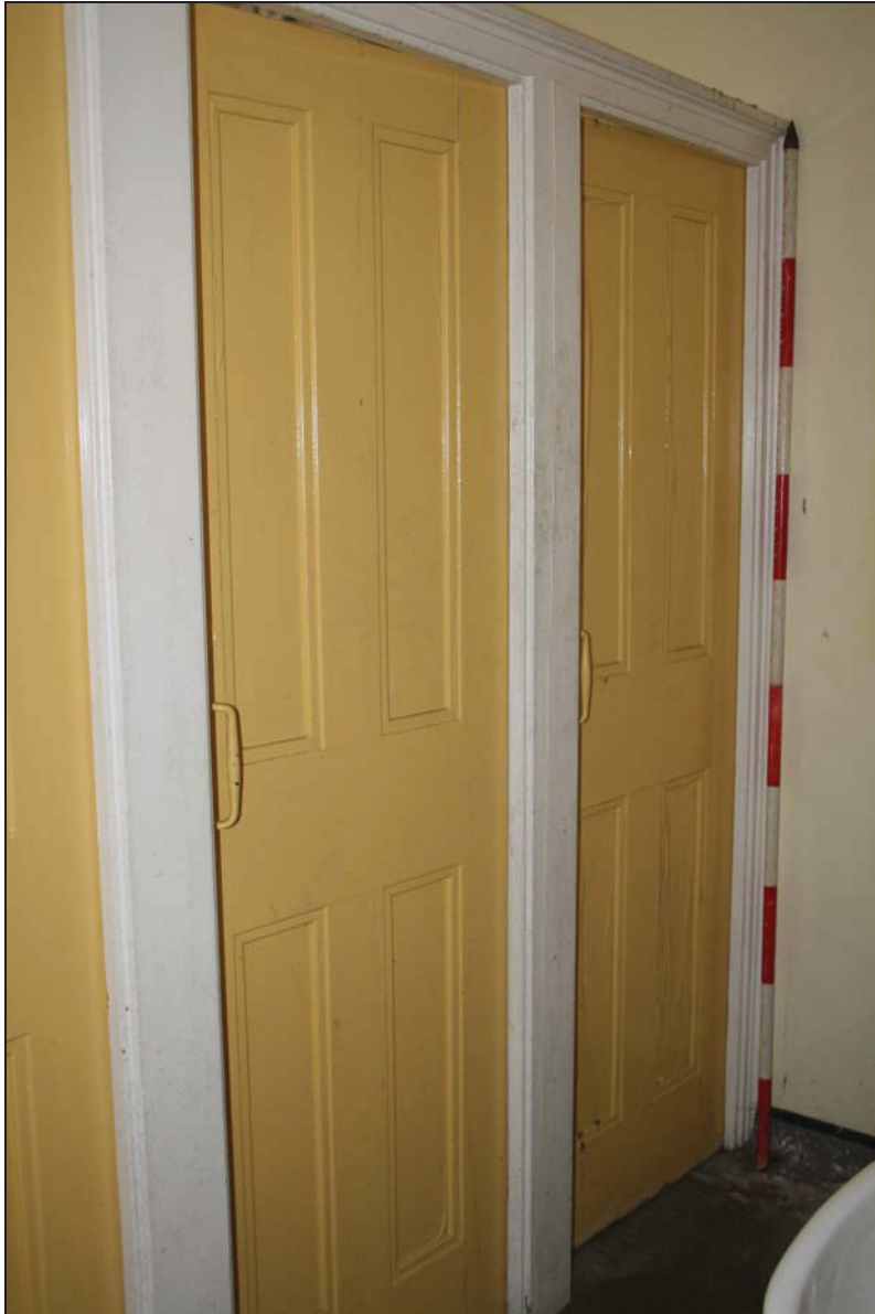
25 Original doors in Room SF03 (Law Building), taken from the south-east (72)
