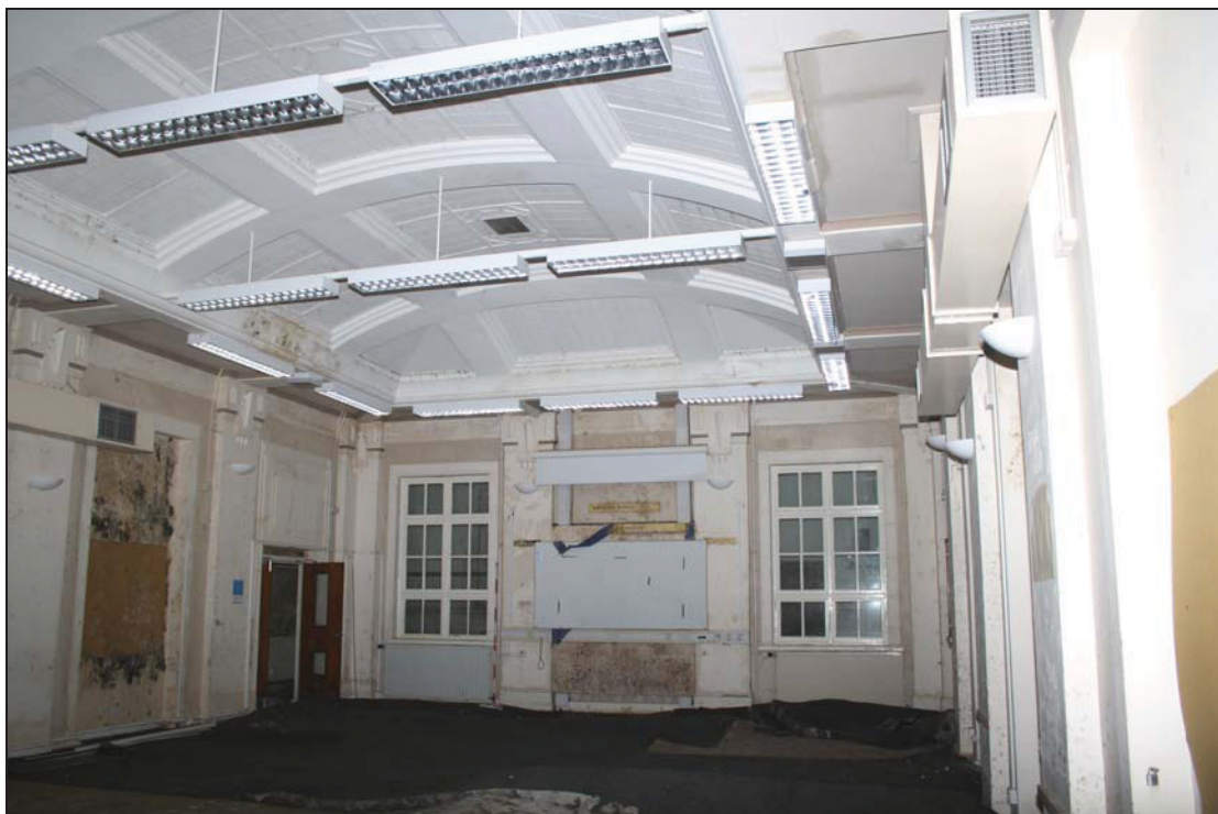
21 Room GF10 (Law Building), taken from the east (46)
