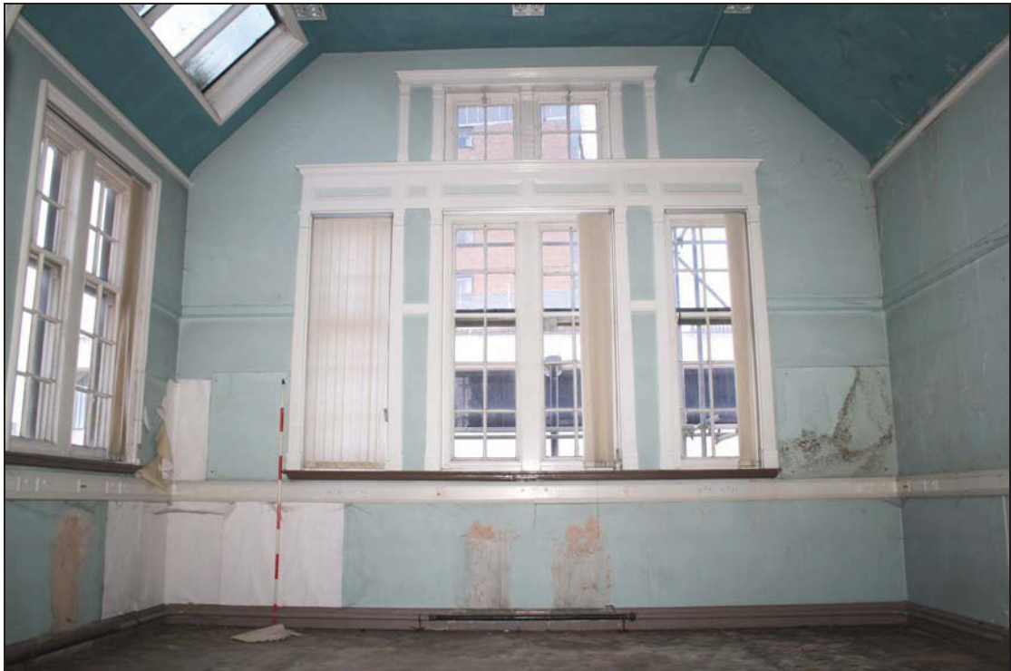
13 Room FF09 (Frederick Chancellor Building), taken from the west (105)
