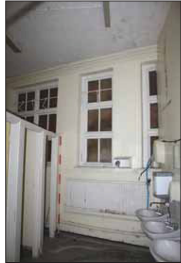
37 Room GF02b (Law Building), taken from the east
