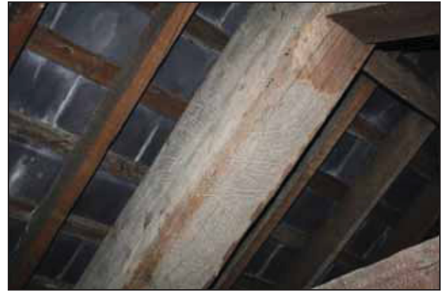
Baltic batch mark on a principal rafter in the roof (Anne Knight Building), taken from the south-east
