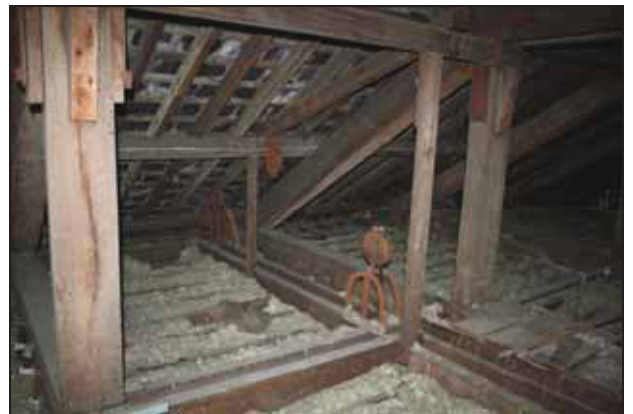
Mechanism in the roof space for a moveable partition which formerly lay below (Anne Knight Building), taken from the north-west
