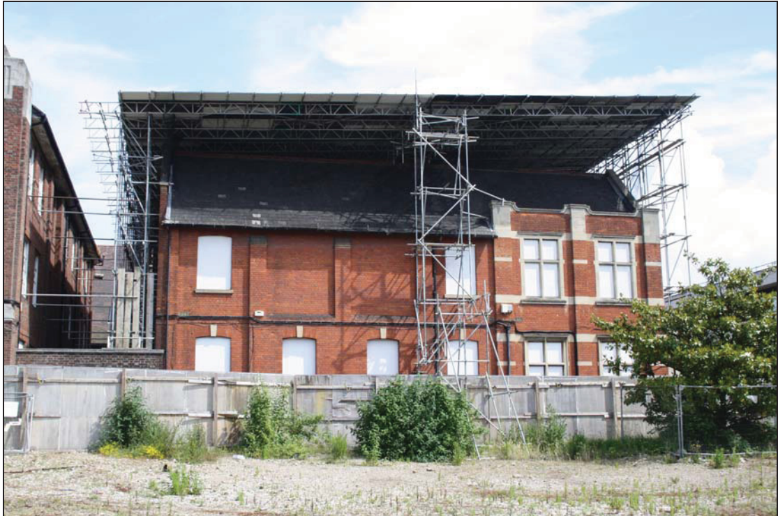
7 South elevation of the Frederick Chancellor Building, taken from the south (12)
