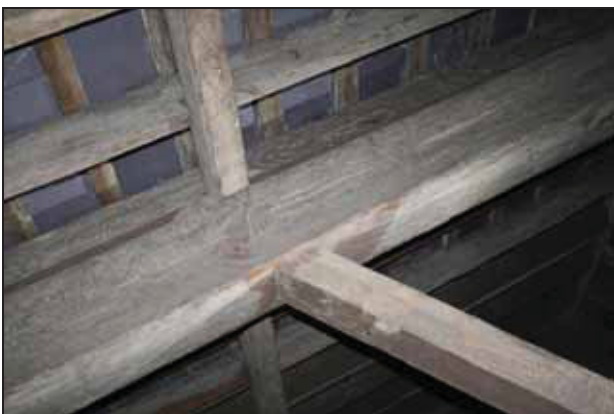
Baltic batch mark on a principal rafter in the roof (Anne Knight Building), taken from the south
