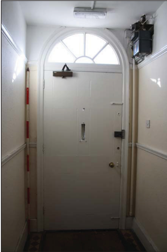
DP 03 Entrance hall (GF01) showing rear face of the doorway, taken from the west
