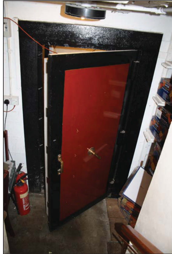
DP 30 Security door to the basement, taken from the north-east
