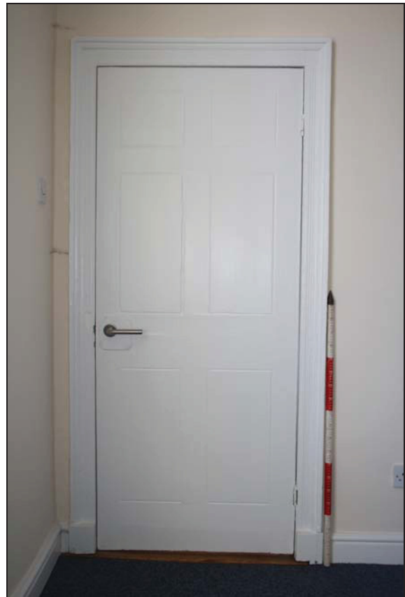
DP 19 Doorway between FF02 and FF03, probably of late 18 th or early 19 th century date with replaced door furniture, taken from the north
