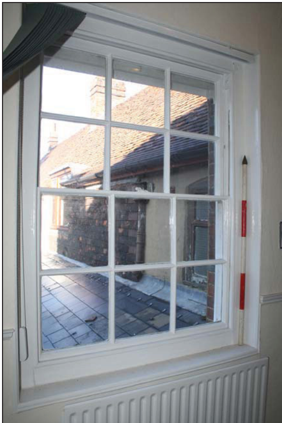
DP 15 18 th or 19 th century sash window lighting the first floor landing (FF01), taken from the south-east
