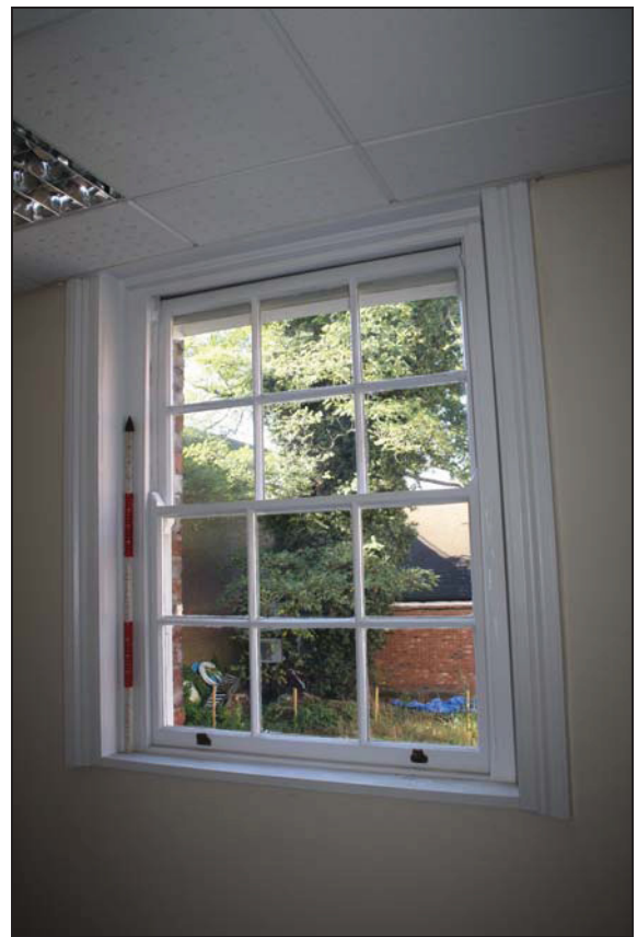
DP 27 Window in Room FF04. 19 th century sashes with some early glass, though the frame has been modified, taken from the north-east
