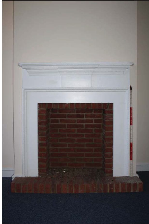
DP 22 Late 18 th century – early 19 th century fireplace in Room FF02, taken from the north
