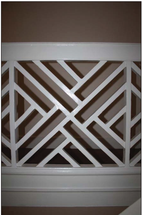
DP 09 Detail of the stair balustrade (FF01), taken from the north
