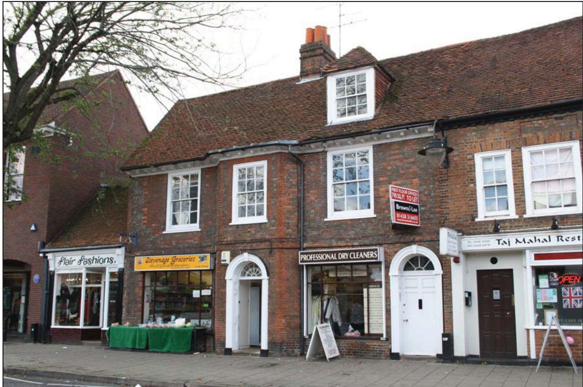
DP 01 Street façade of the assessment building, taken from the east
