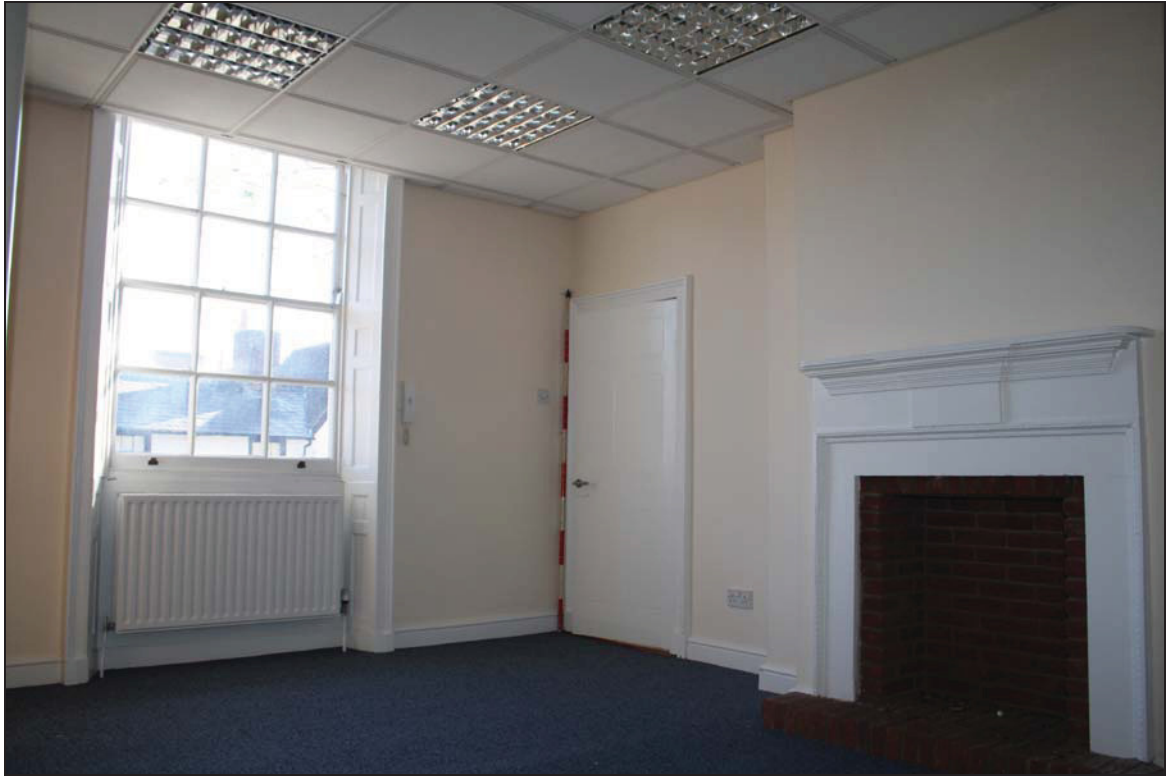
DP 17 First floor room fronting the street which retains a number of early features including the window surround and shutters, doorway and fireplace (FF02), taken from the north-west
