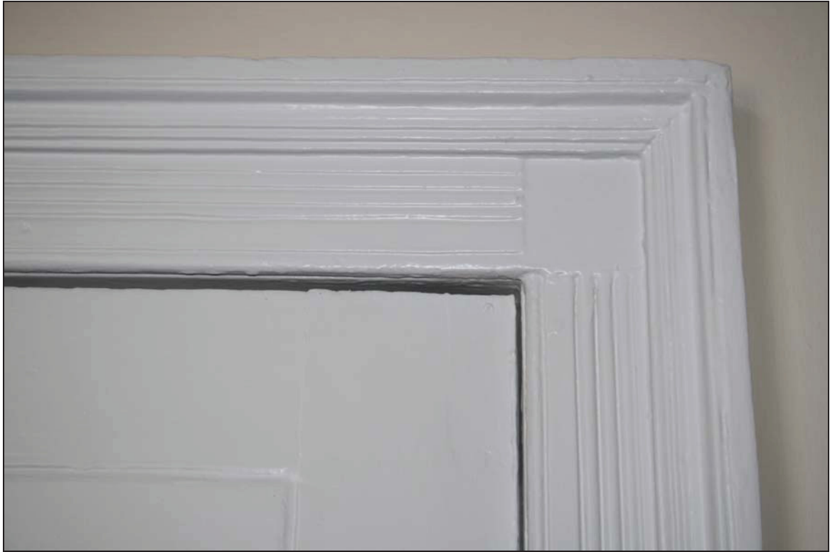
DP 20 Detail of the architrave between Rooms FF02 and FF03 showing reeding and square paterae, taken from the north
