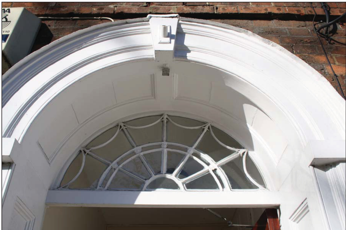
DP 02 Detail of the fanlight over the south doorway, probably late 18 th – early 19 th century in date, taken from the east
