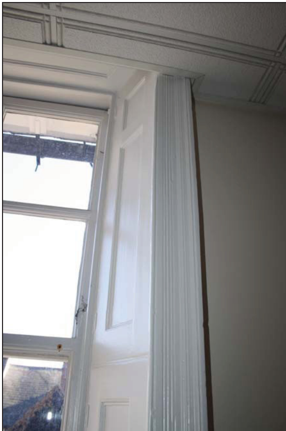
DP 18 Detail showing shutter form and surround (FF02), taken from the west
