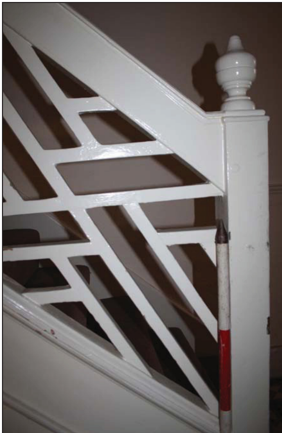
DP 08 Detail of the stair balustrade (GF02), taken from the south
