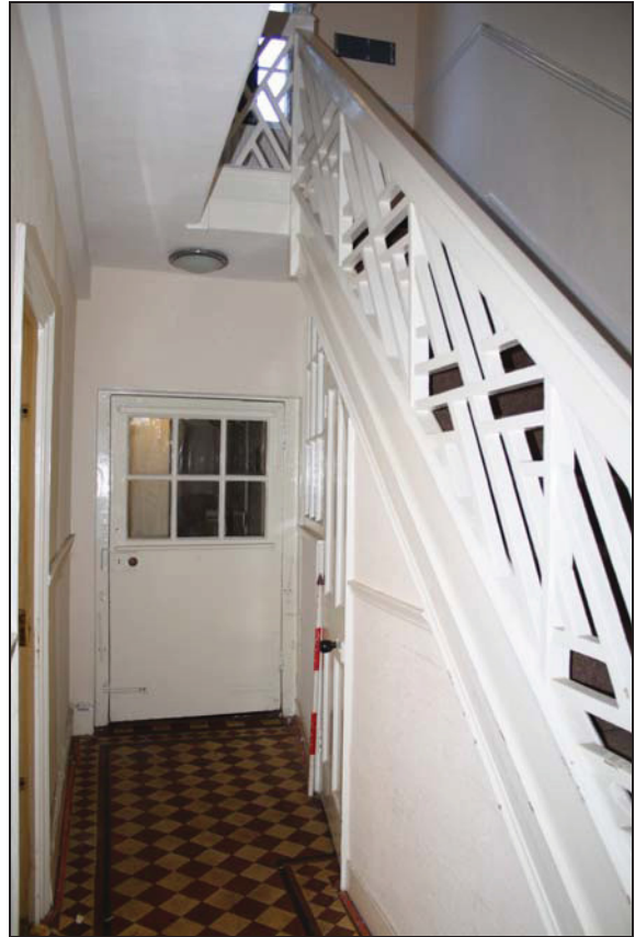
DP 07 Stair vestibule (GF02) showing original back door, taken from the east
