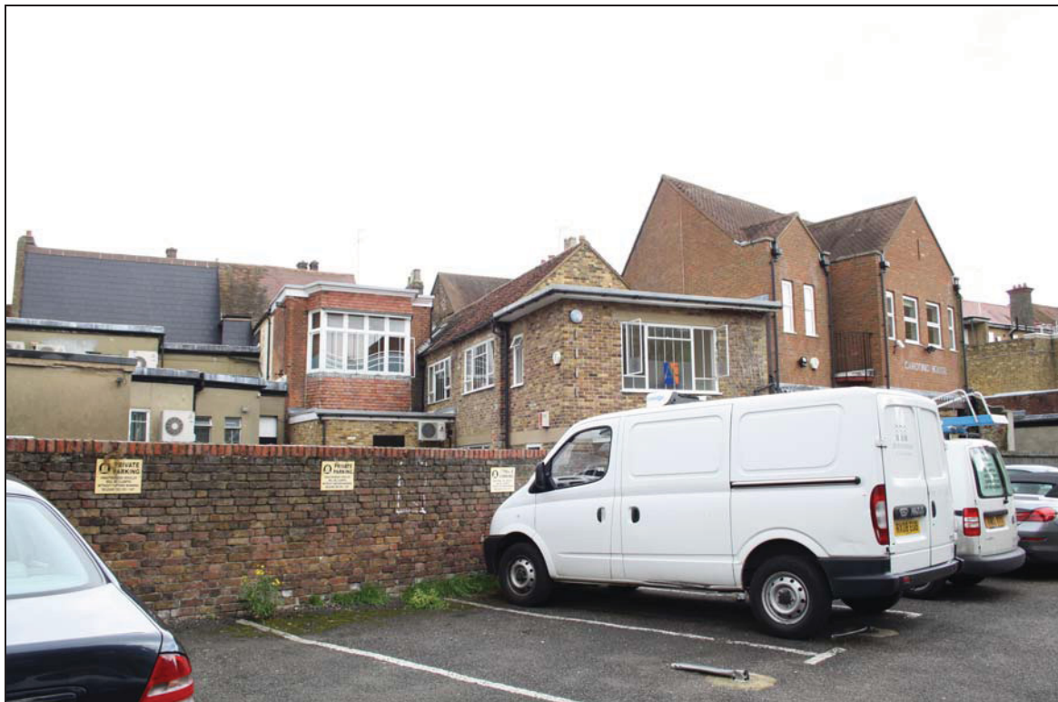
Plate 2 View of the rear ranges of No. 127 and flanking buildings, taken from the south-west (DP 01)
