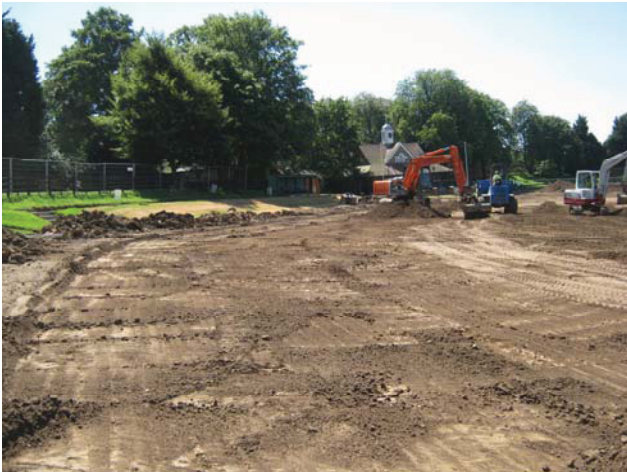
DP 3. Eastern part of the site. Looking south.
