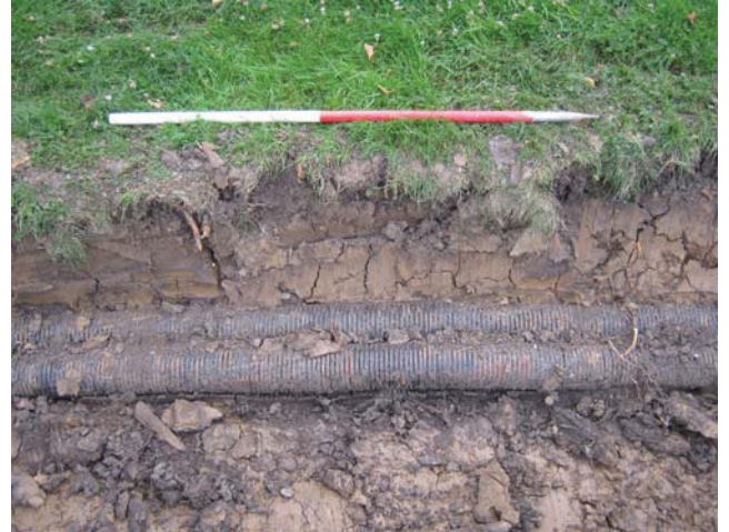
DP 8. Service trench. Sample section 1.
