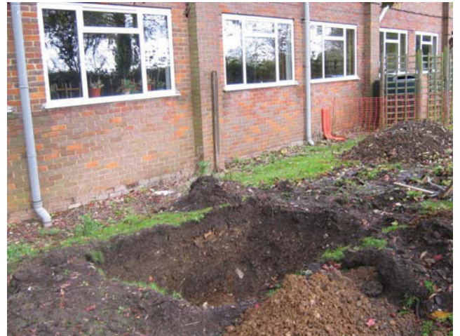
DP 2. Test Pit 1. Looking north-east.
