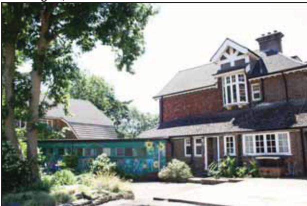
71 East side of Building B with linking corridor, taken from the east
