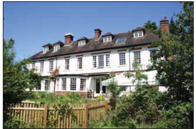
42 South elevation of Building X2, taken from the south-east
