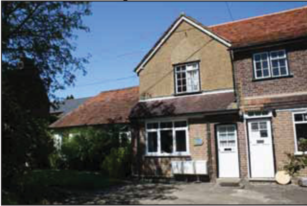
65 South side of Building F, taken from the south-east
