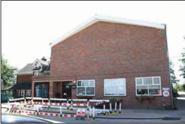
97 East side of Building A, taken from the east
