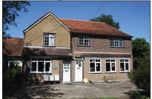
64 South side of Building F, taken from the south
