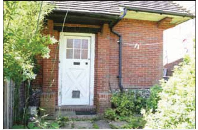
68 East side of Building Q, taken from the east
