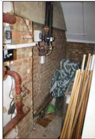
94 Exposed brick construction of Building A at basement level
