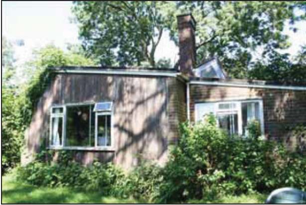
37 South side of Building X4, taken from the south
