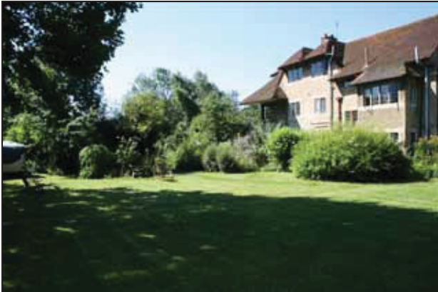
27 East side of Building M (west range, south end) and lawn area, taken from the north-east
