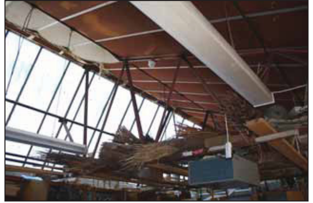
98 Roof structure of Building E, taken from the west
