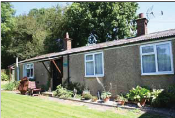
47 West side of Building O, taken from the south-west
