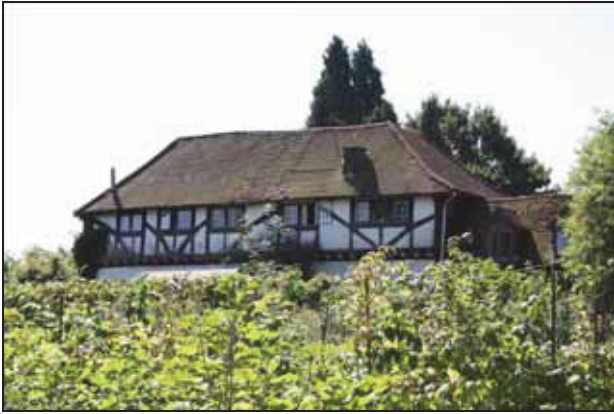
25 North side of Building M (north range), taken from the north
