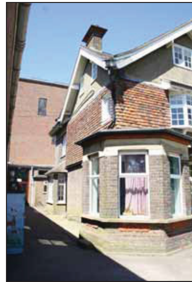
76 West side of Building B, taken from the south
