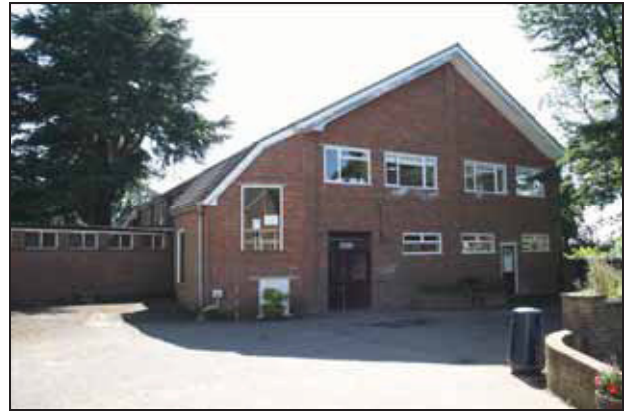
14 West elevation of Building C, taken from the west
