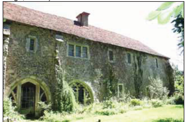
60 West elevation of Building M, taken from the west
