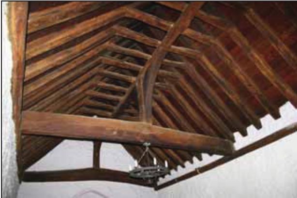
57 View of the crown-post roof within Building M (west range, centre)
