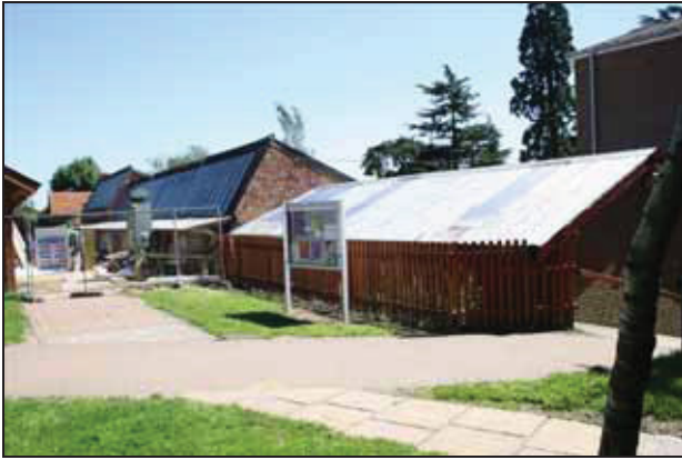
61 North side of Building E, taken from the north-west
