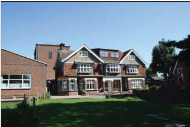
15 View of Building B with Building A on the left, taken from the south
