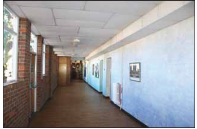
74 Ground floor corridor space in Building C, taken from the west
