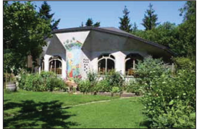
46 View of Building K, taken from the south
