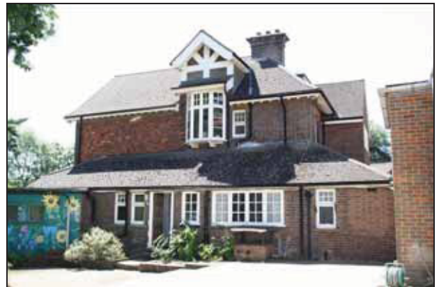
72 East side of Building B, taken from the east
