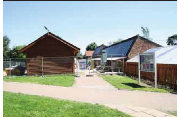
62 West side of Buildings N and E, taken from the west
