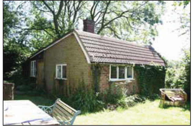
38 North and west sides of Building X4, taken from the north-west
