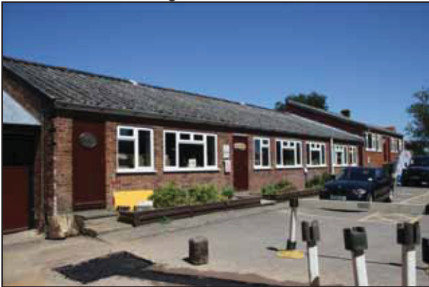
63 South side of Building E, taken from the south-west
