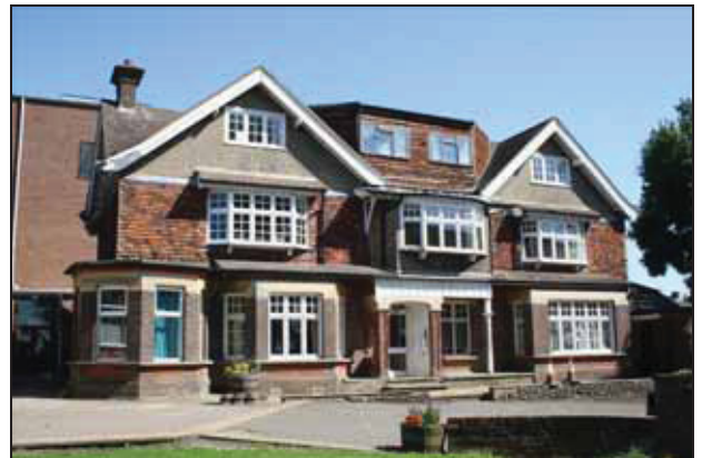
16 South elevation of Building B, taken from the south
