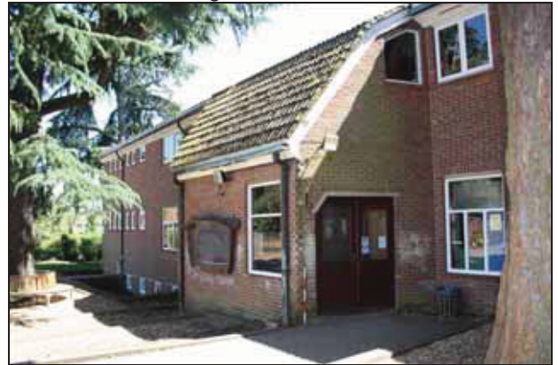
70 North side of Building C, taken from the north-west
