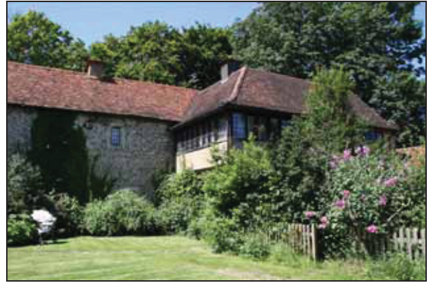
56 East side of Building M (west range, north end), taken from the south-east
