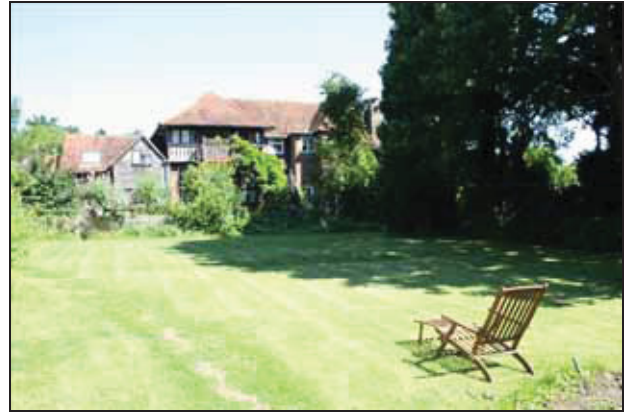
26 South side of Building M (north range) with lawn area, taken from the south
