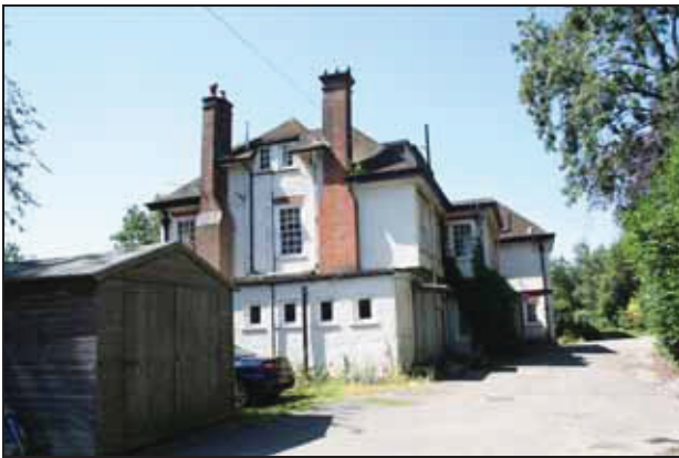
41 East elevation of Building X2, taken from the east
