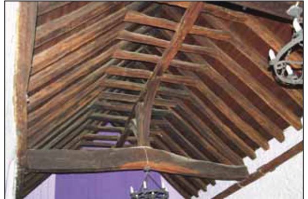
58 View of the crown-post roof within Building M (west range, centre)
