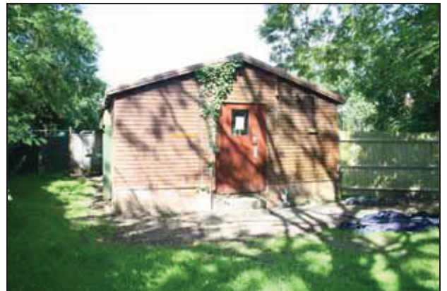
12 View of Building G, taken from the east
