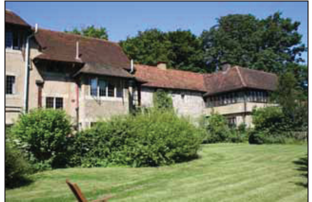
28 East side of Building M (west range, north end), taken from the south-east
