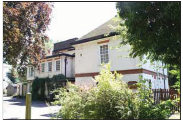
40 North elevation of Building X2, taken from the north-west
