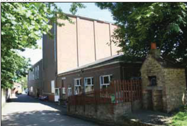
95 North side of Building A, taken from the west
