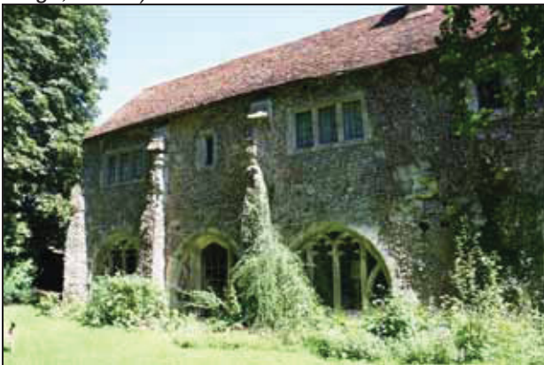
59 West elevation of Building M, taken from the west
