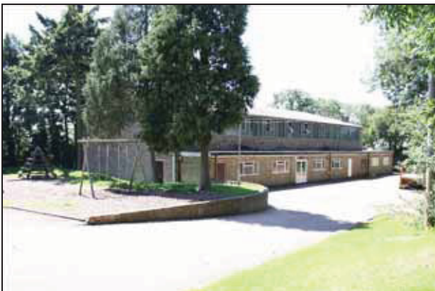
53 Northern side of Building H, taken from the north-east
