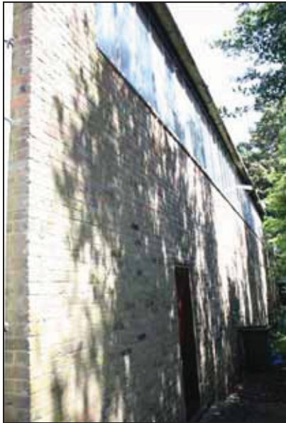
51 South side of Building H, taken from the west
