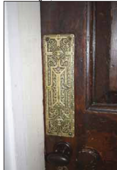
78 Example of brass finger-plate on a door in Building B, taken from the east
