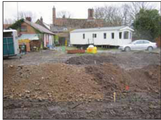
2 General view of site. Looking south towards rear of Hunston House.
