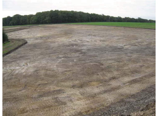
DP 2. Area G1. Looking south.
