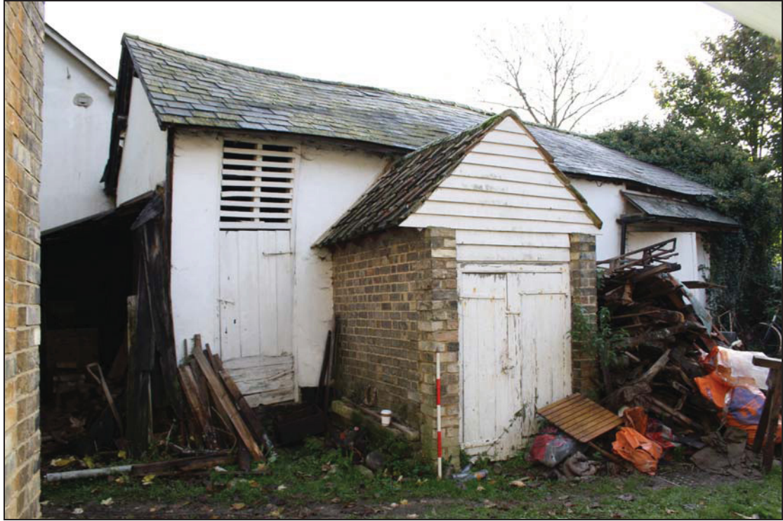
Plate 13 West elevation, Range 2, taken from the north-west (DP 50)
