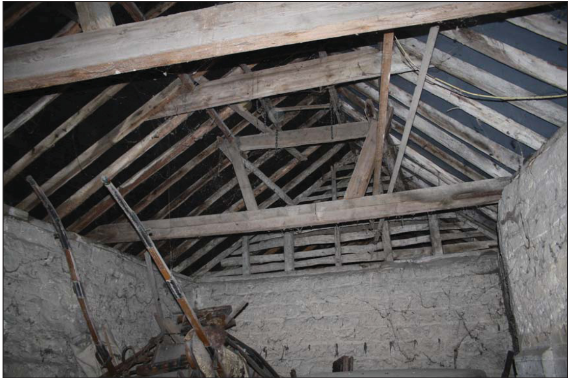
Plate 14 Roof above Unit 2, Range 2, taken from the south-east (DP 83)
