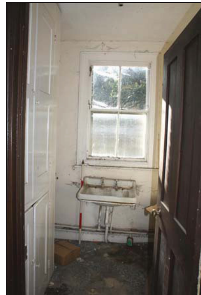
22 Room FF07, taken from the north
