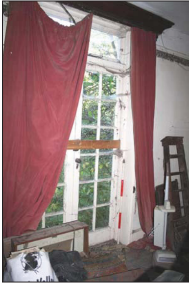
19 French doors in Room GF06, taken from the south-east
