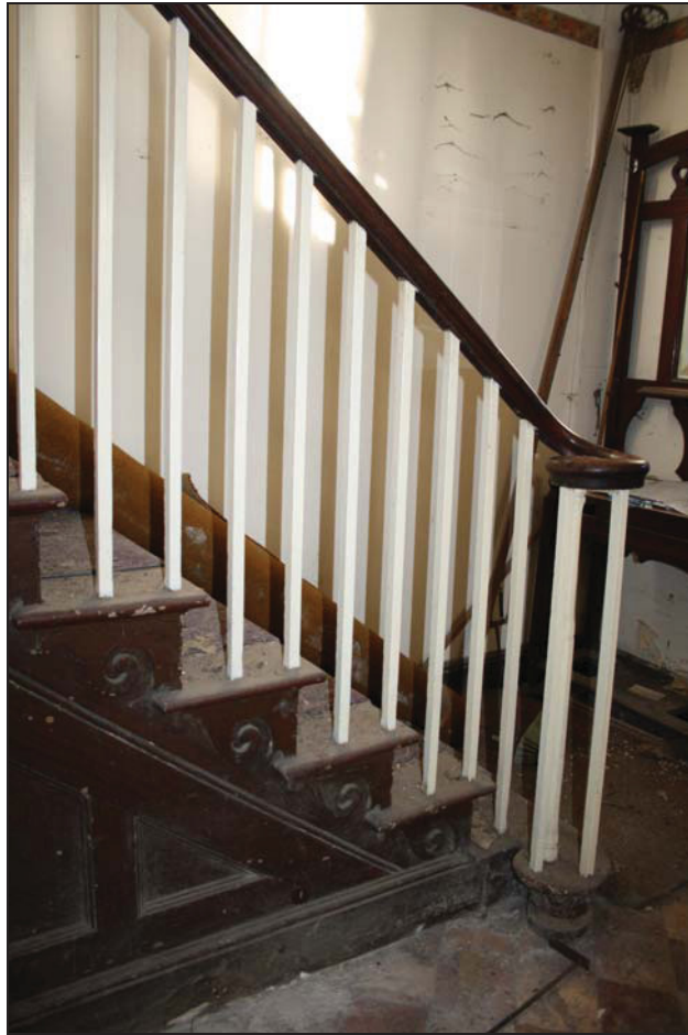
Plate 3 Staircase, GF02, taken from the south-east (DP 10)
