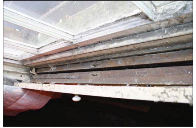
Vertically sliding shutters housed within the window apron in Room GF03, taken from the south-east
