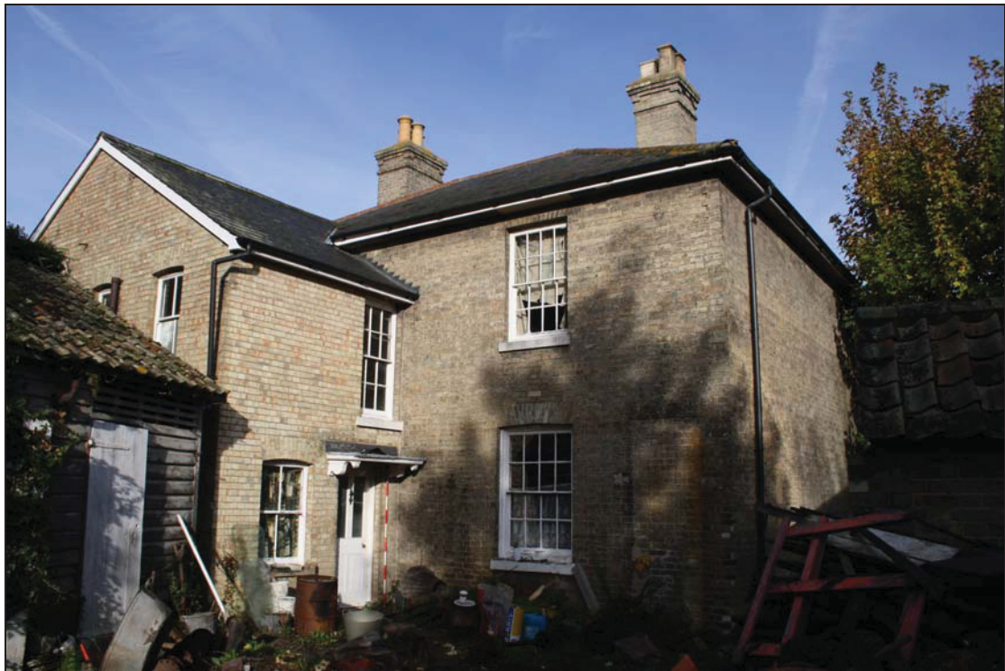
Plate 2 Farmhouse, rear elevation, taken from the south-east (DP 40)
