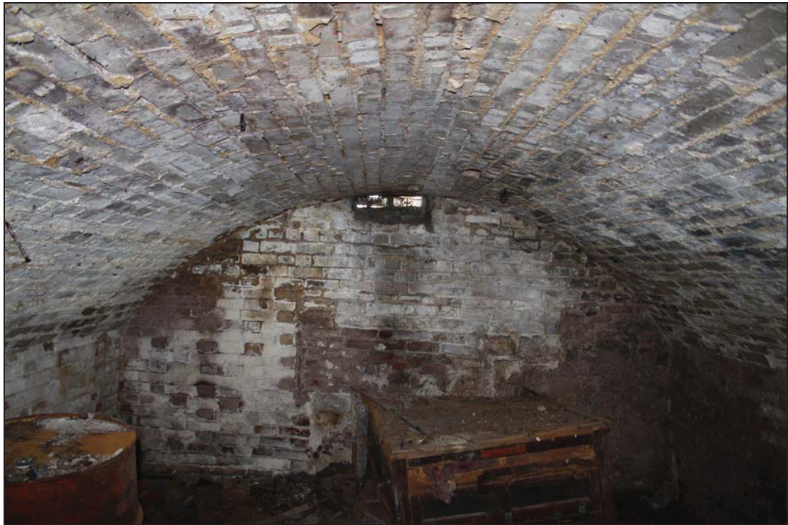
Plate 15 Barrel vaulted cellar beneath Range 2, taken from the north-west (DP 69)
