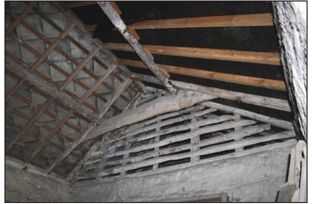
Timber-framed upper gable in Unit 1, Range 2, taken from the north-west
