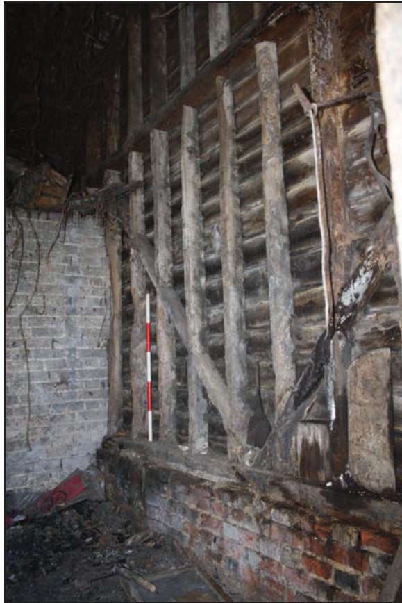
Plate 11 North elevation of Unit 1, Range 1, taken from the east (DP 71)
