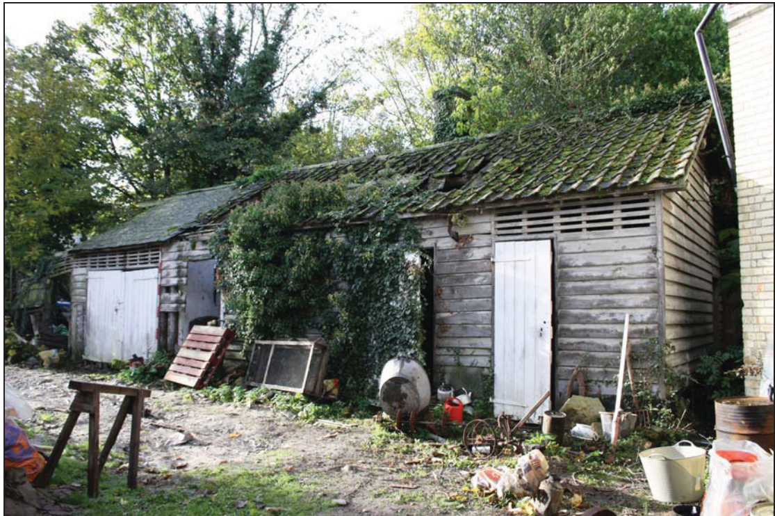
Plate 10 East elevation, Range 1, taken from the north-east (DP 48)
