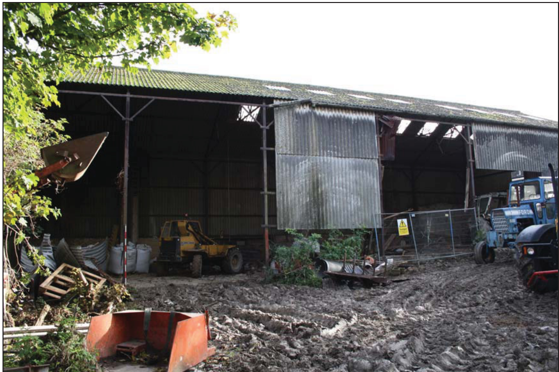
Plate 18 Open-fronted west elevation, Range 5, taken from the north-west (DP 53)
