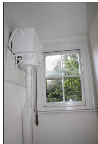
24 Room FF08, taken from the north
