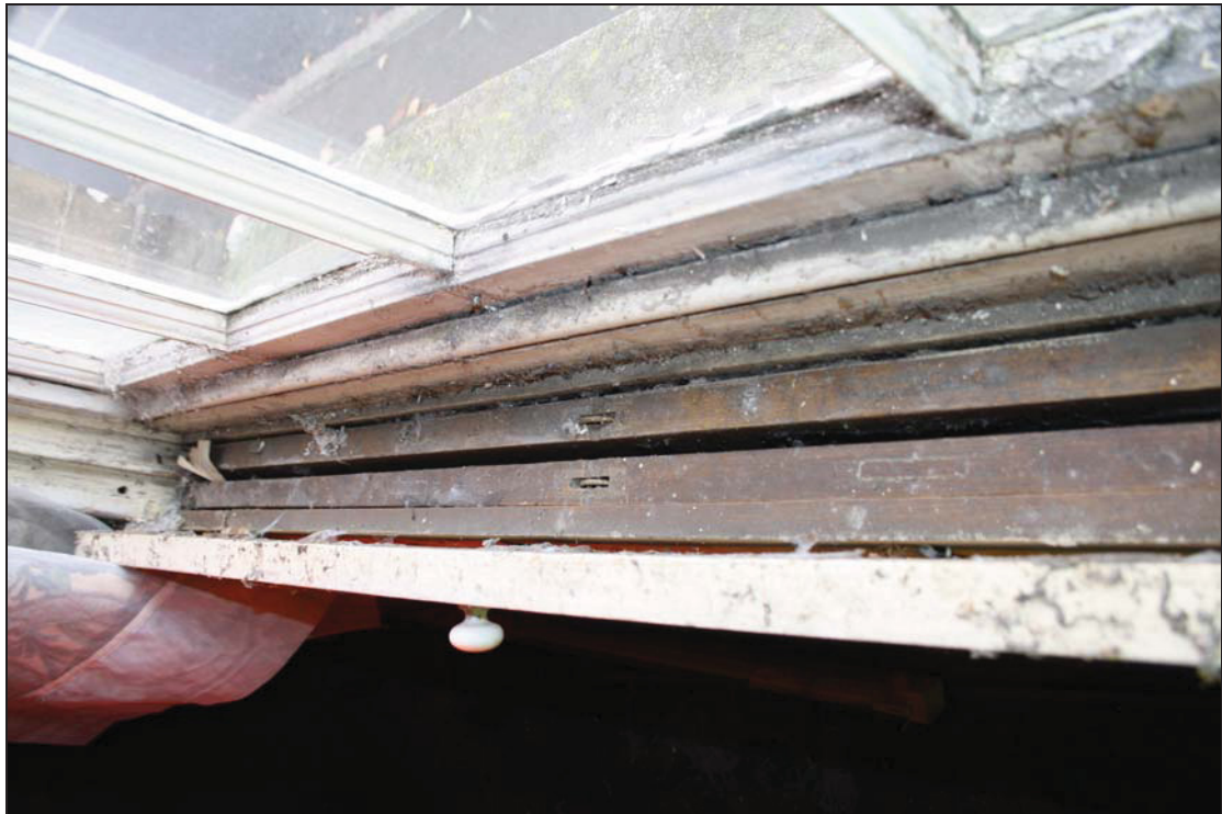
Plate 4 Vertically sliding shutters housed within the window apron in Room GF03, taken from the south-east (DP 38)
