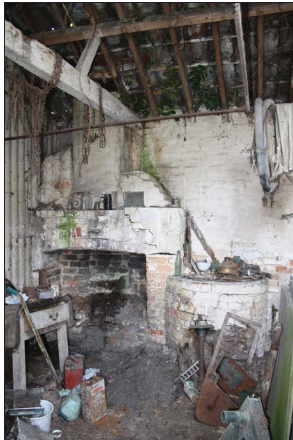
Plate 12 Fireplace and copper in Unit 2, Range 1, taken from the east (DP 82)
