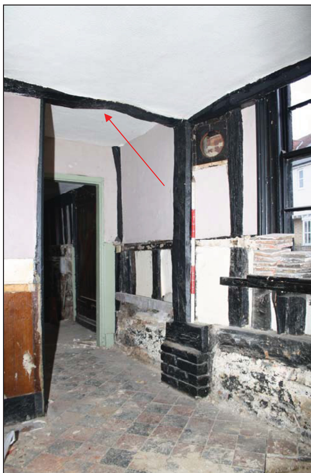
Plate 5 Junction between Room GF01 and the lobby on the south side of the chimney stack with curved notch in the soffit (indicated), taken from the north-west (15)
