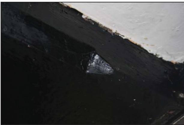
Chamfer-stop at the east end of the binding joist in Room GF04, taken from the east
