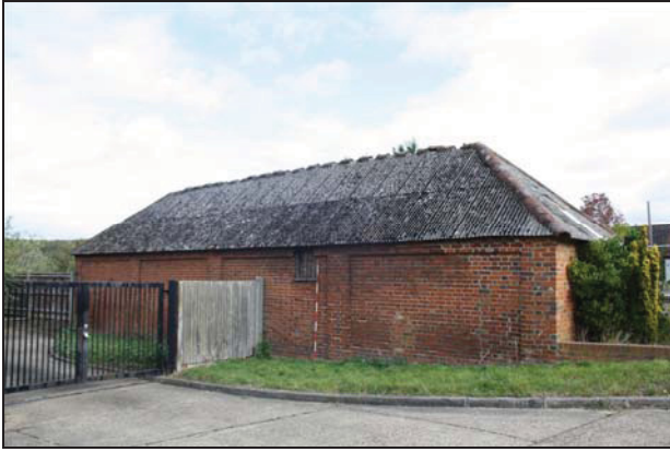
West elevation of outbuilding showing blind panels and southern reconstruction, taken from the south-west
