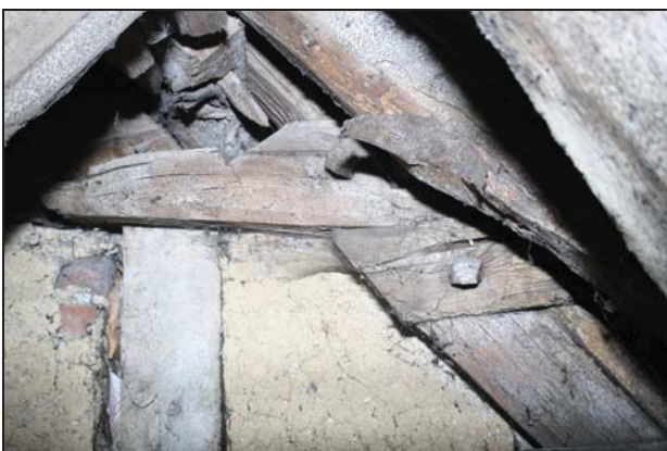
53 Detail of the rafter and collar to the west of the chimney stack, taken from the east
