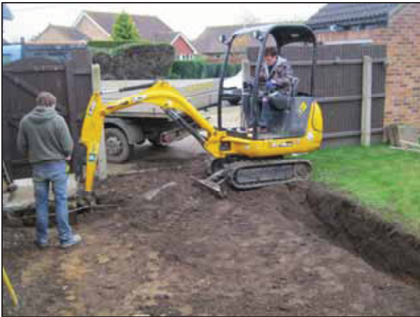
Footing trench excavation in progress. Looking southeast.
